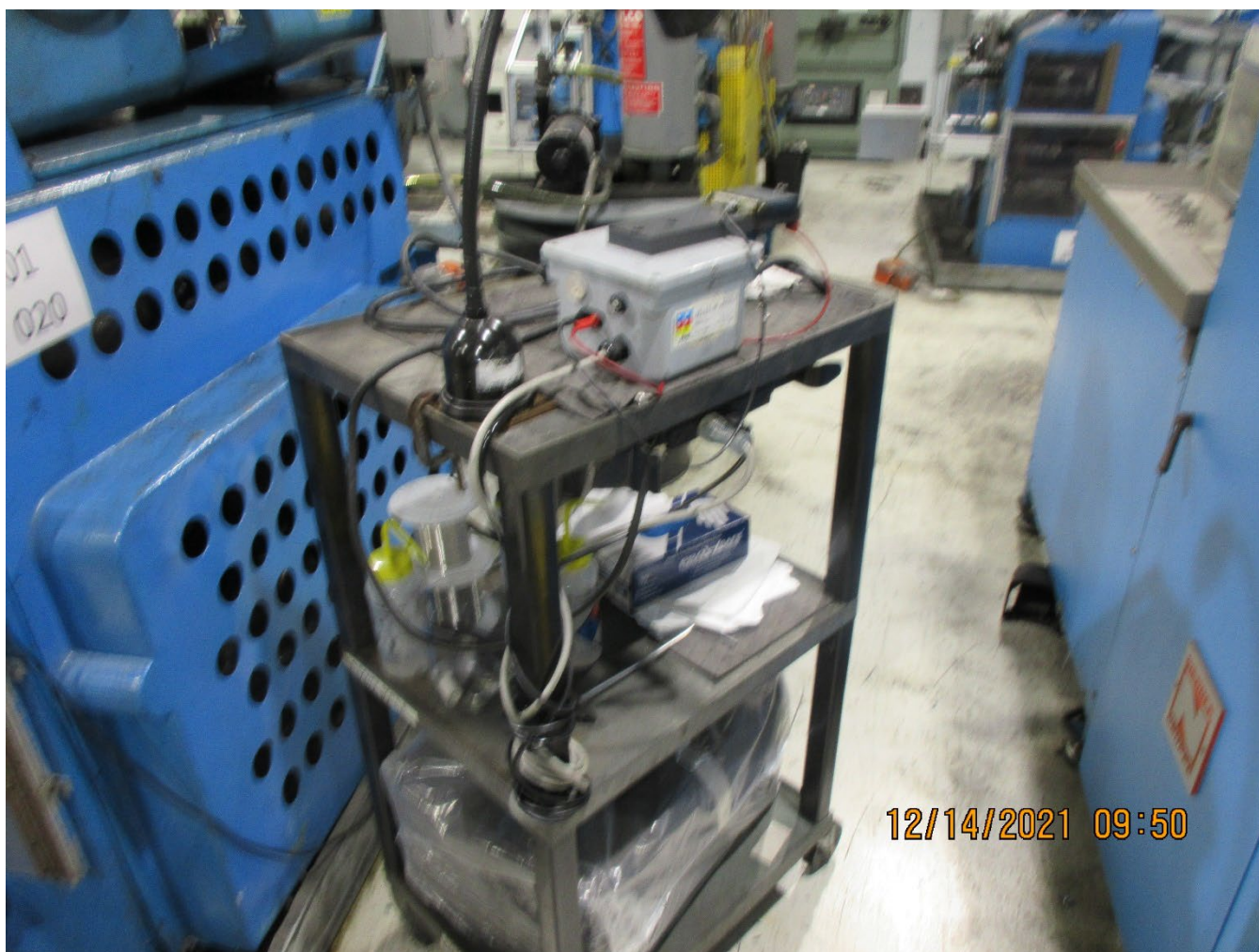
Photo 2 - Commerce 3 Acid Pot on Cart in Main Room
