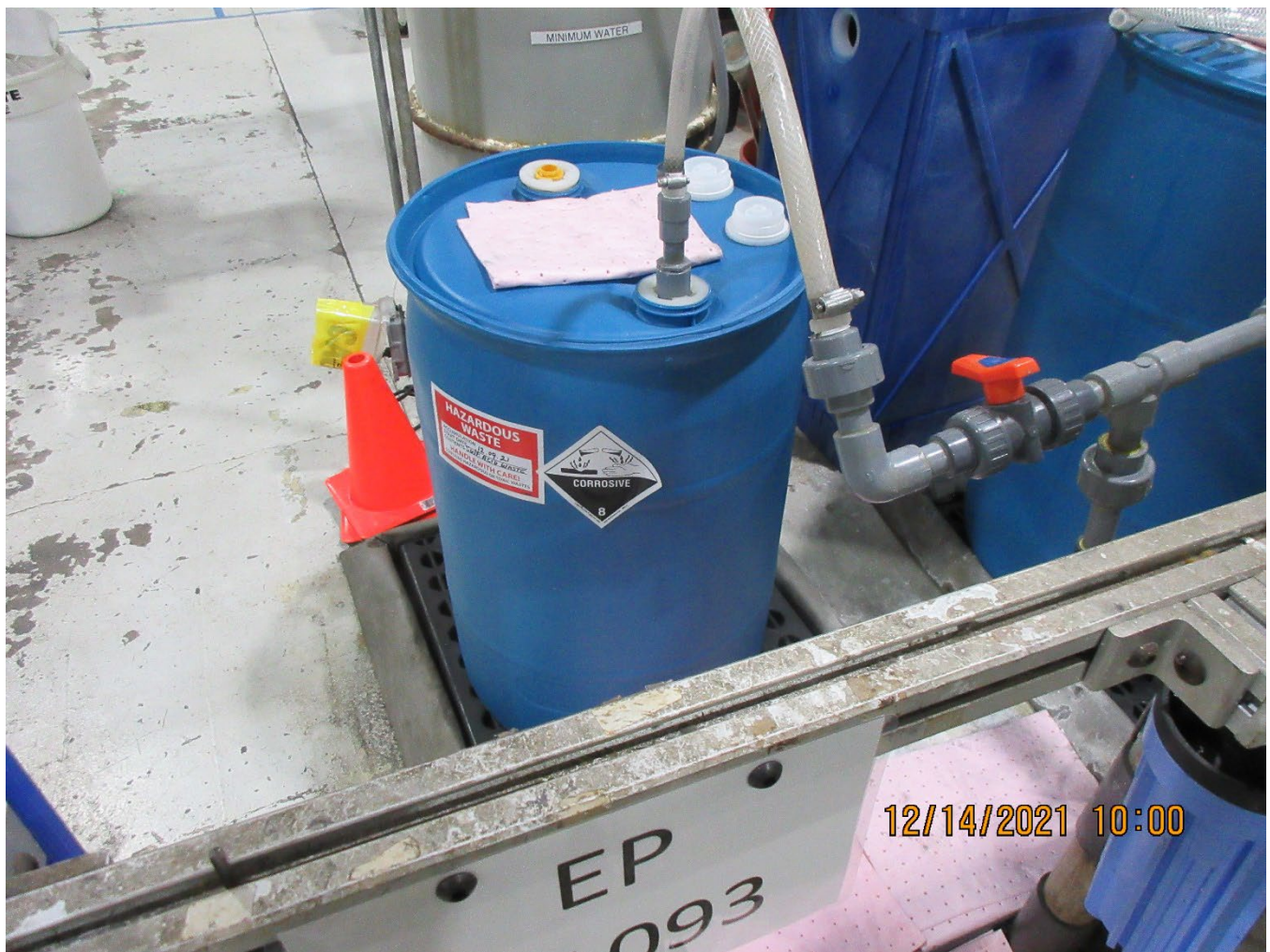
Photo 4 – Commerce 3 30-gallon drum for spent acid from the electropolishing line in the Main Room
