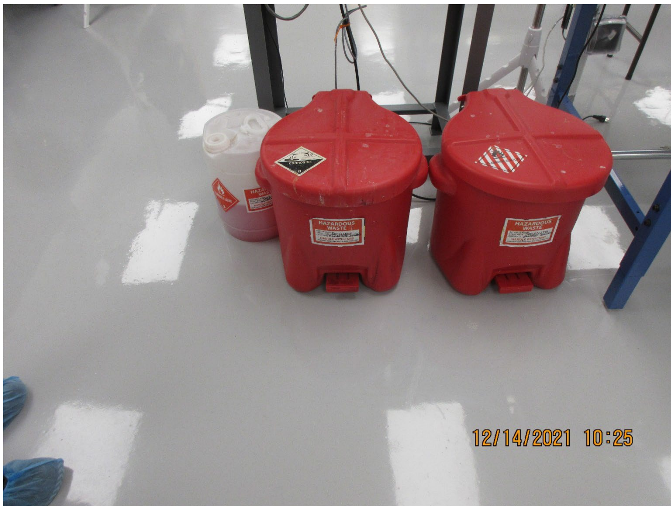
Photo 10 – Commerce 3 Satellite Accumulation Area within Components Room
