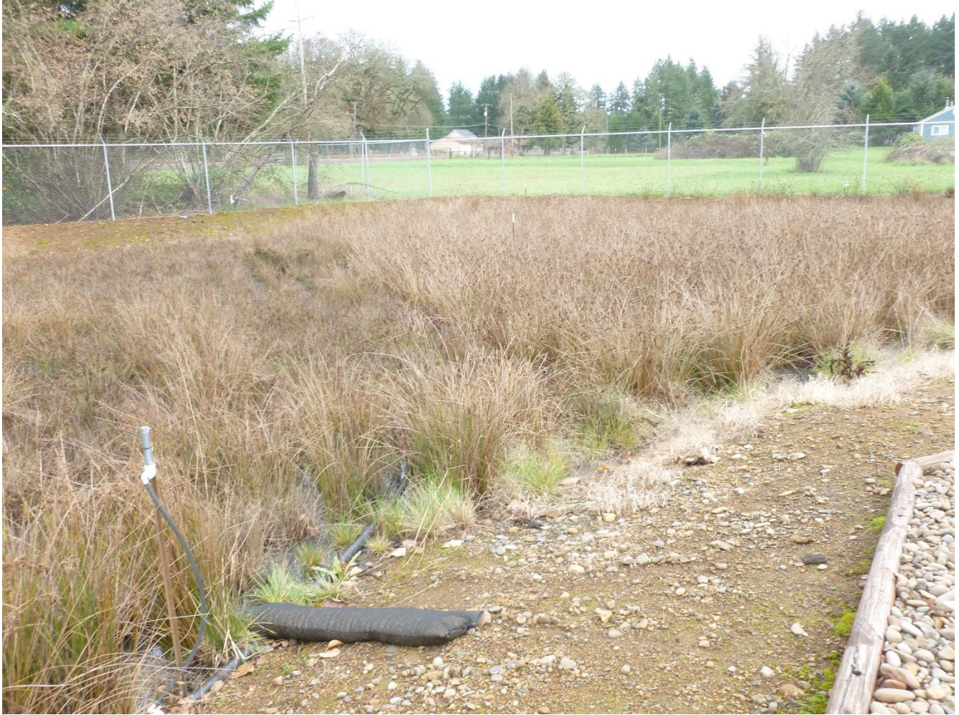
Photo 17 / P1010110 – Bioswale, photo 2
