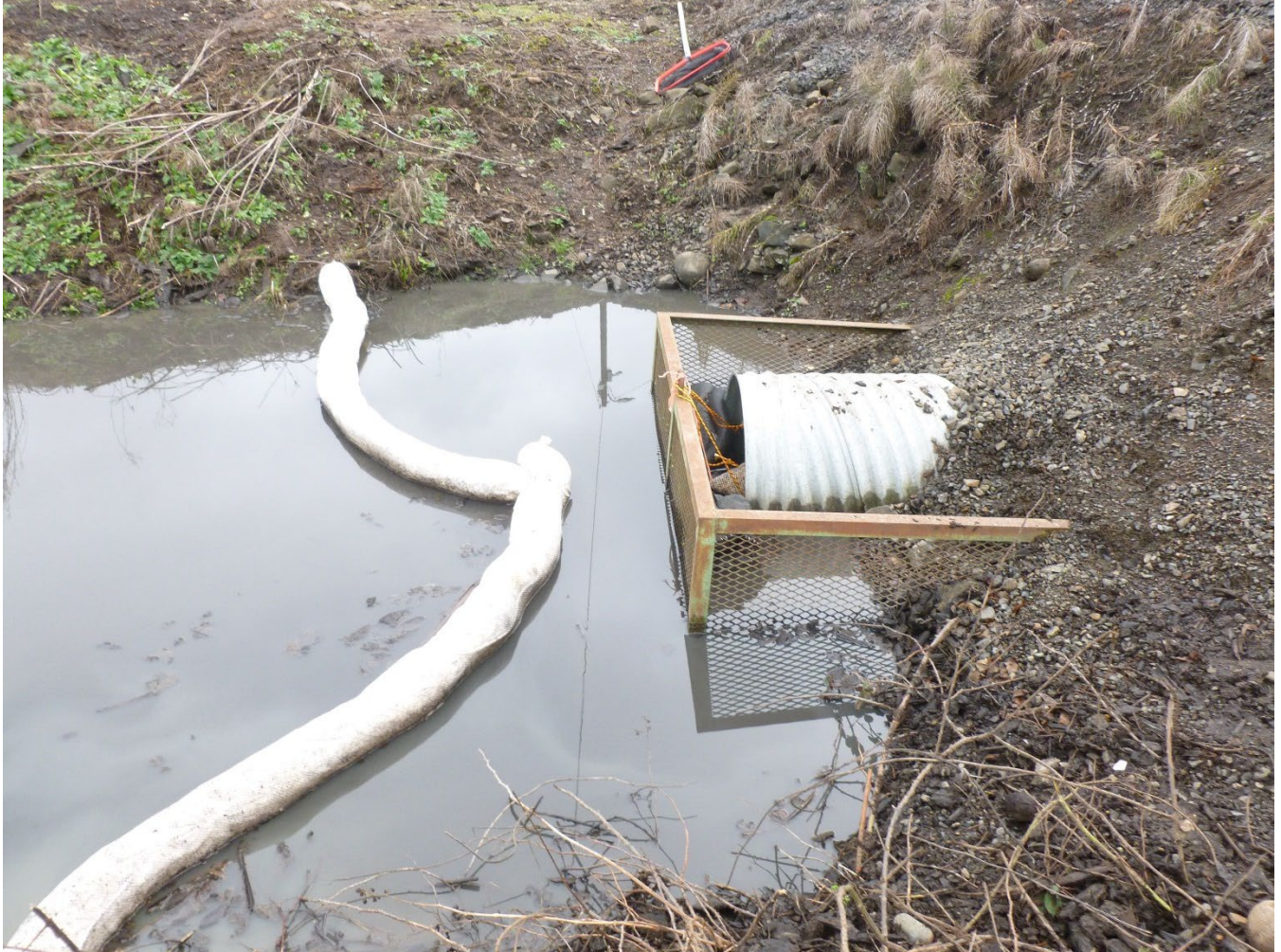
Photo 18 / P1010111 – Monitoring Point 001
