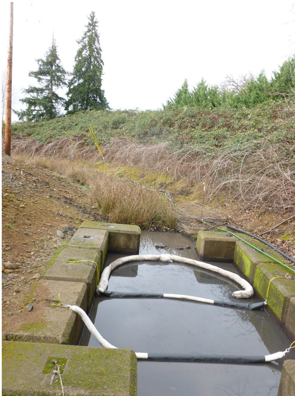
Photo 14 / P1010107 – Settling Basin, photo 3
