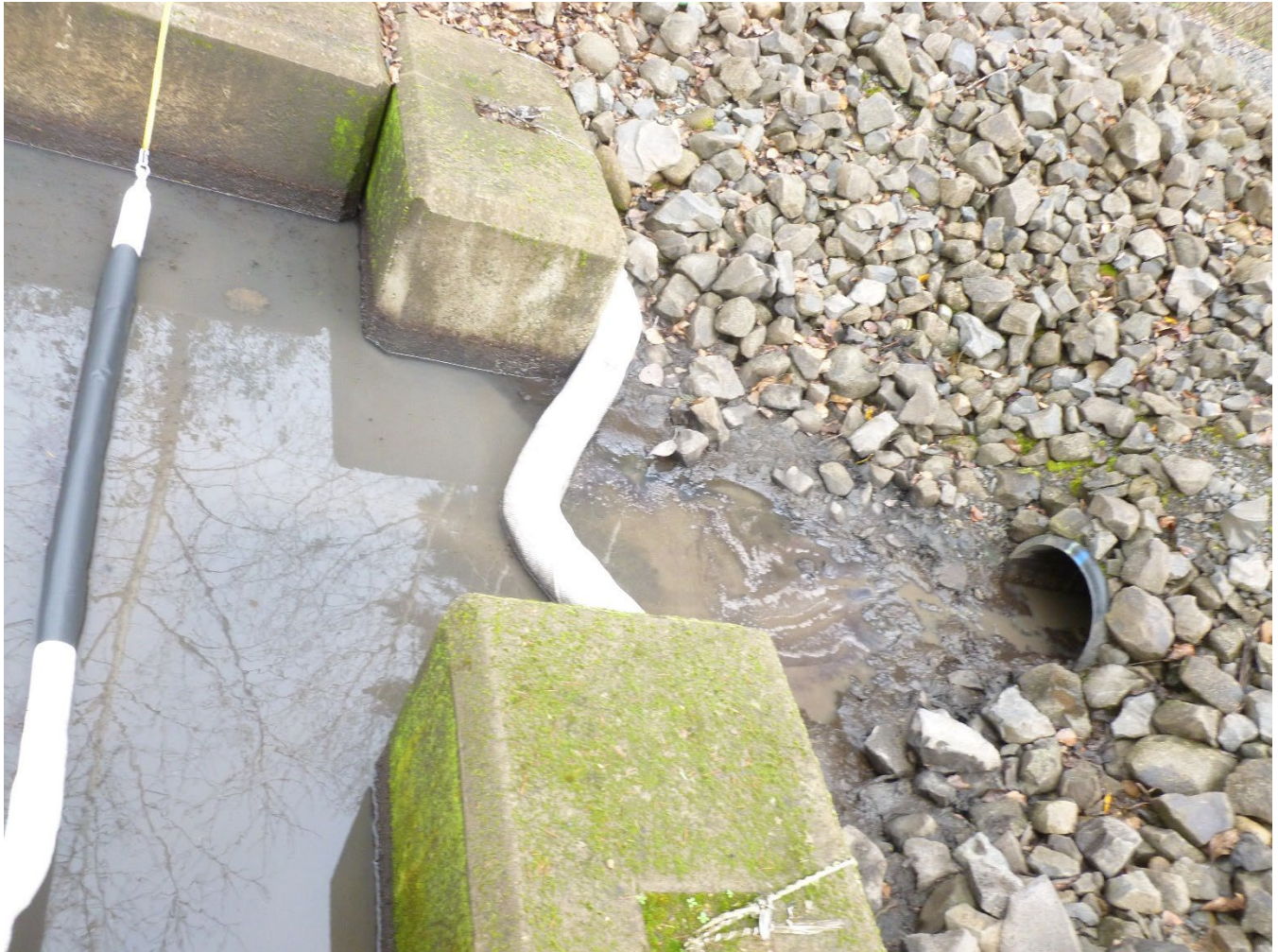
Photo 12 / P1010105 – Settling Basin, photo 1
