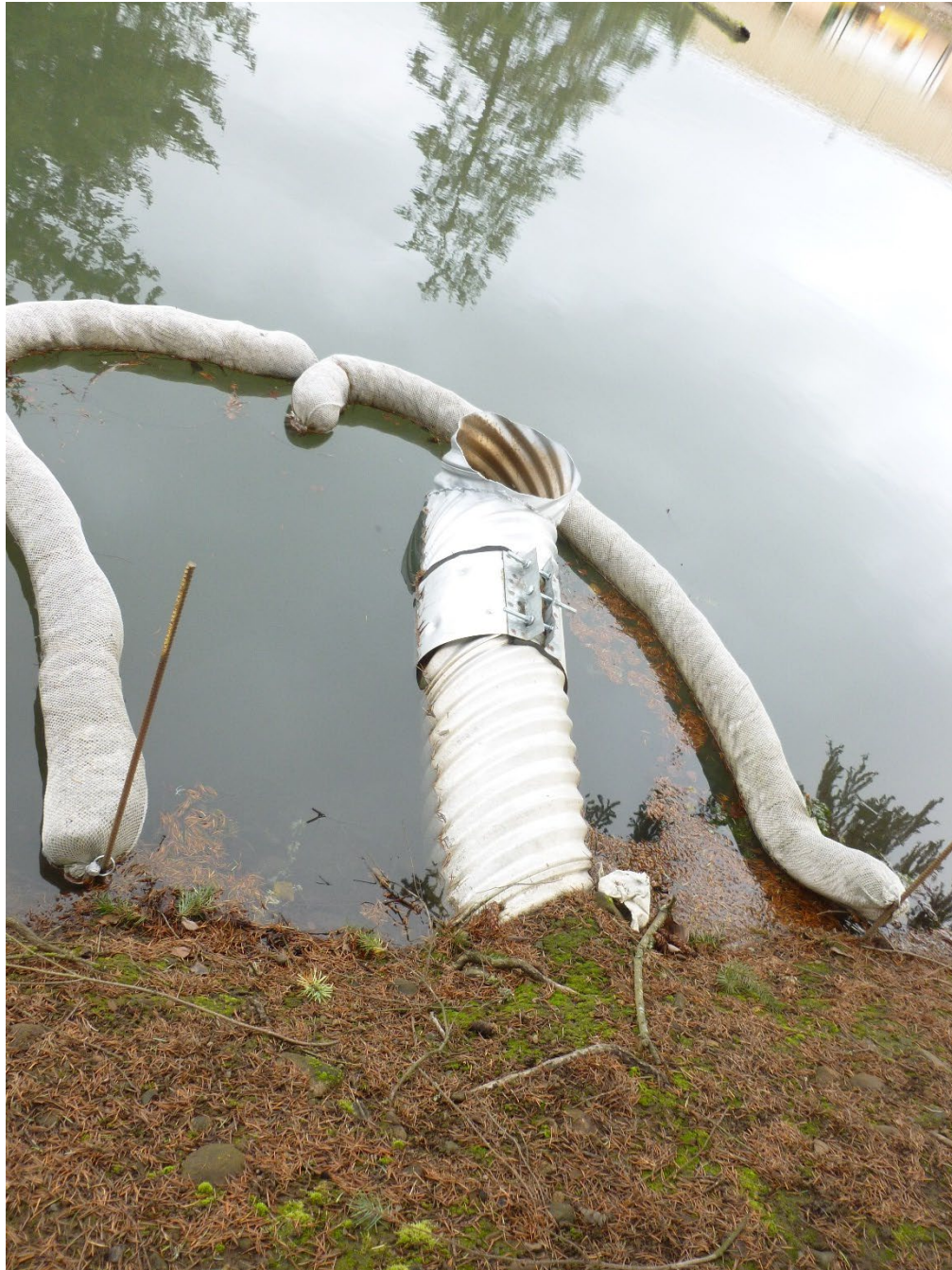
Photo 7 / P1010101 – Fire Pond Overflow, close-up
