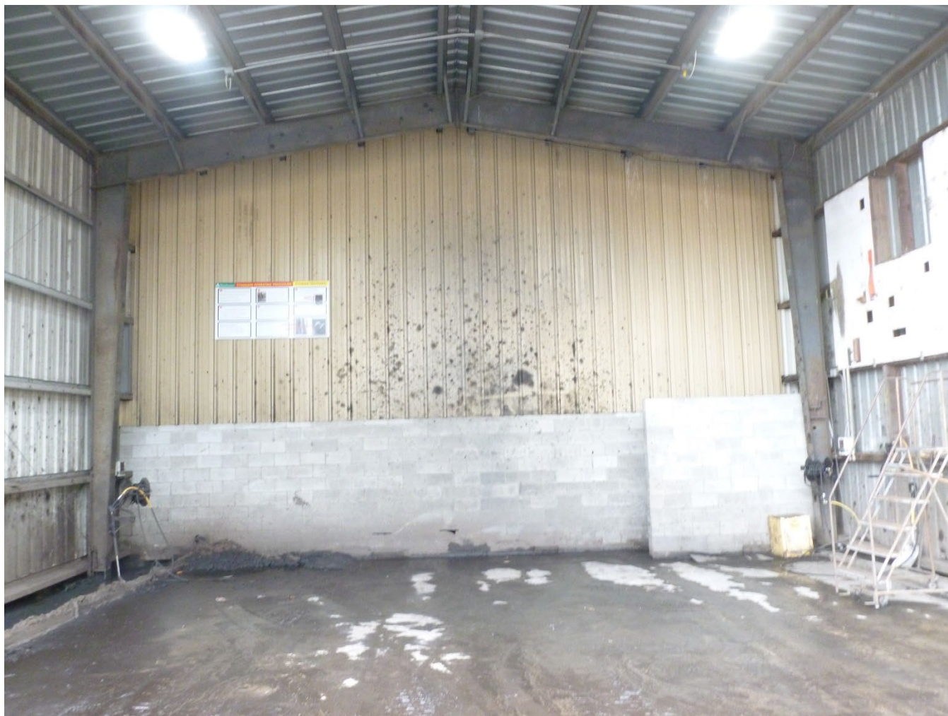
Photo 1 / P1010091 – Truck Wash Bay
