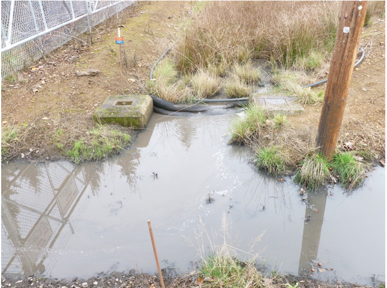
Photo 15 / P1010108 – Monitoring Point 005
