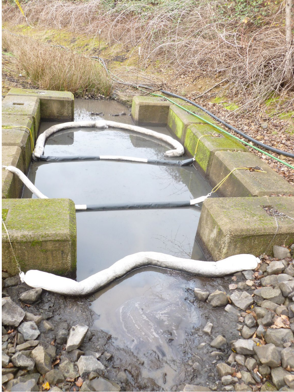
Photo 13 / P1010106 – Settling Basin, photo 2
