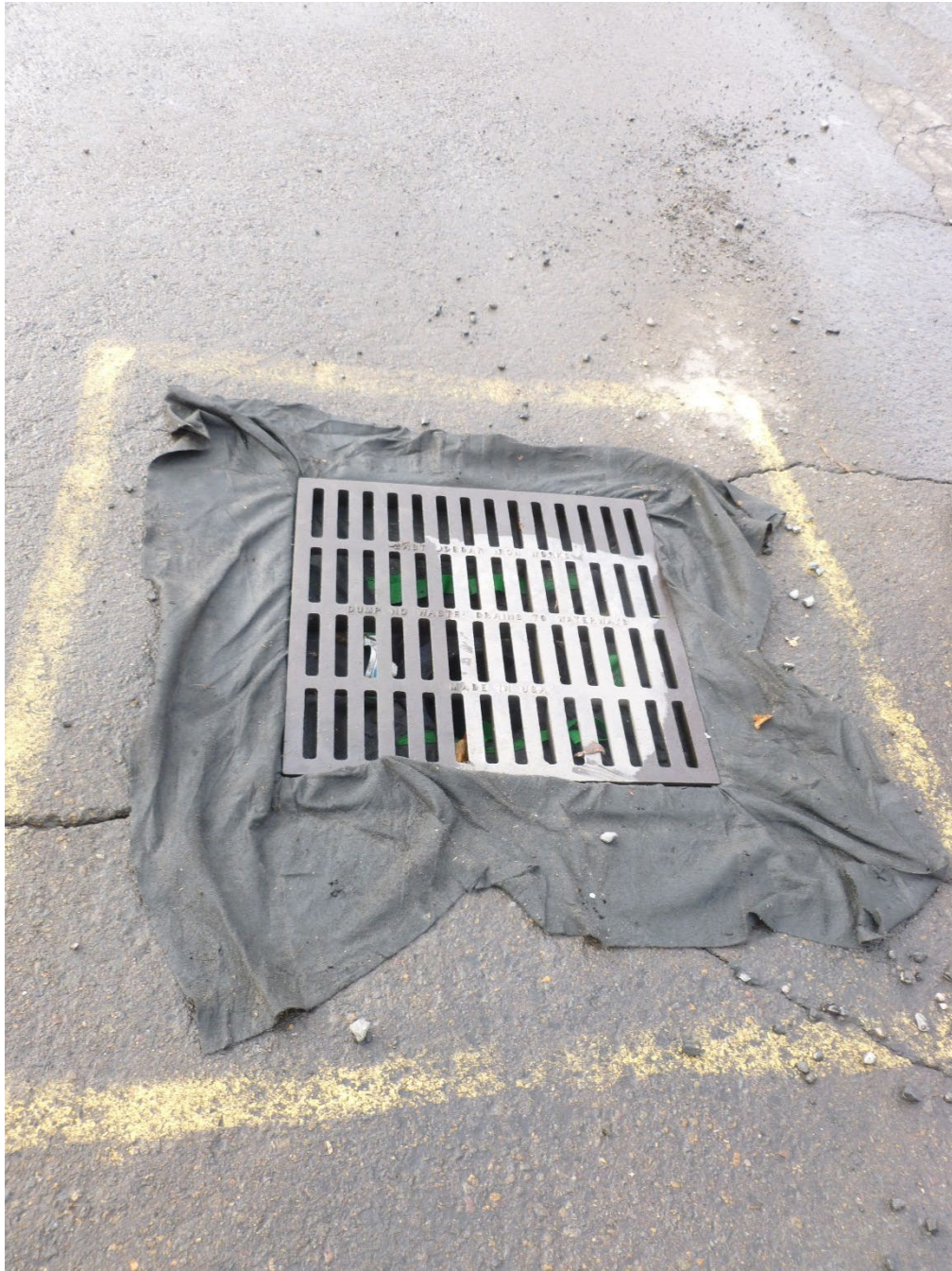
Photo 4 / P1010094 – Catch Basin/Monitoring Point 006, close-up
