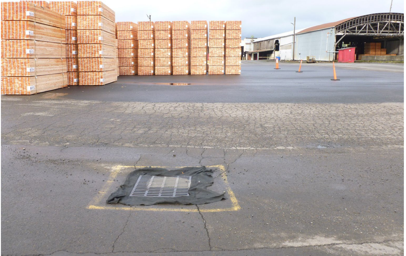
Photo 3 / P1010093 – Catch Basin/Monitoring Point 006
