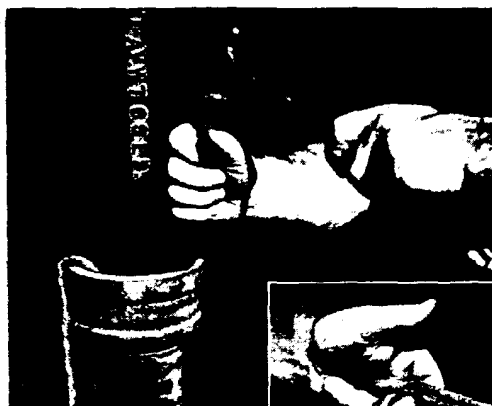
When two lengths of lead wool are joined in a joint, the end of each rope is reduced to half its thickness and the ends overlapped and rolled together avoiding a bulge
