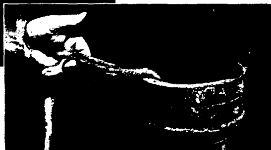
When two lengths of lead wool are joined in a joint, the end of each rope is reduced to half its thickness and the ends overlapped and rolled together avoiding a bulge
