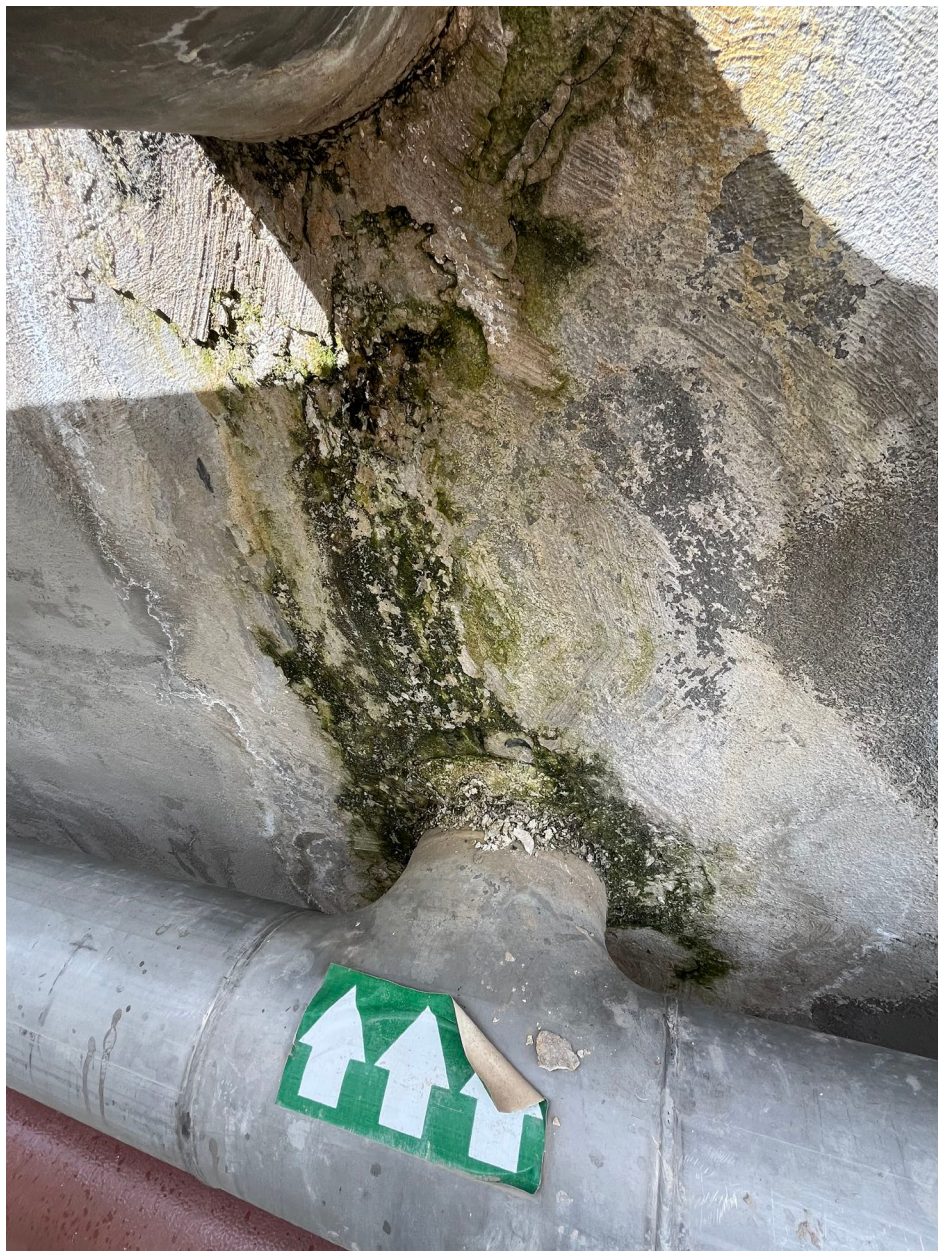
Close-up view of the same air piping penetrations identified in Photo No. 6 above. (IMG_0324). 03/27/2025 11:36 AM Photographed by D. Esparza
