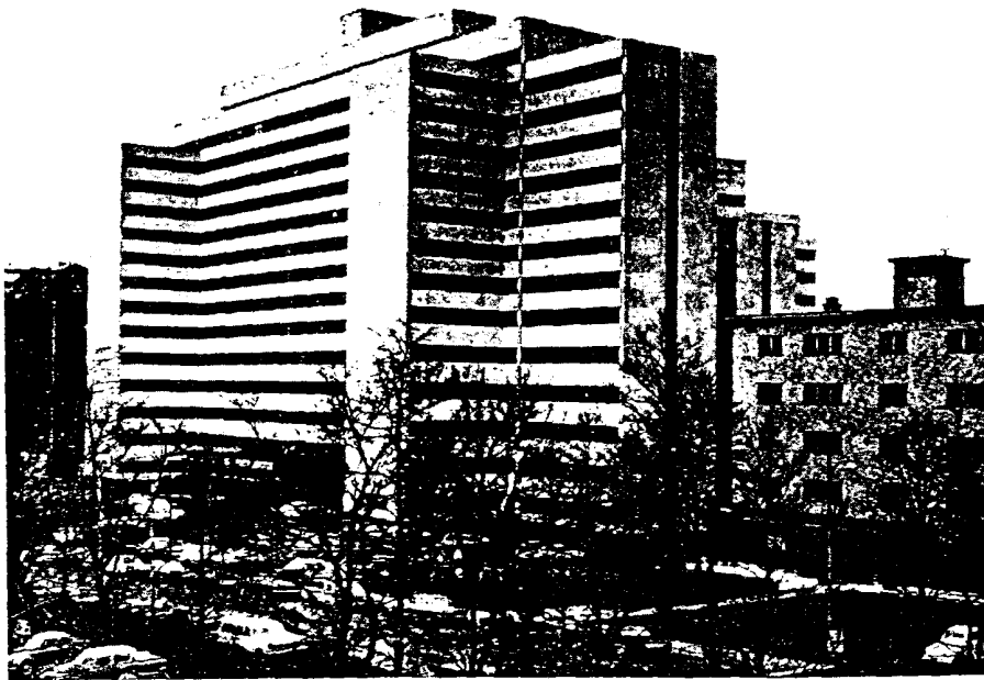
Panel Fabricator: Plasteel Products Corp. Washington, Pennsylvania
