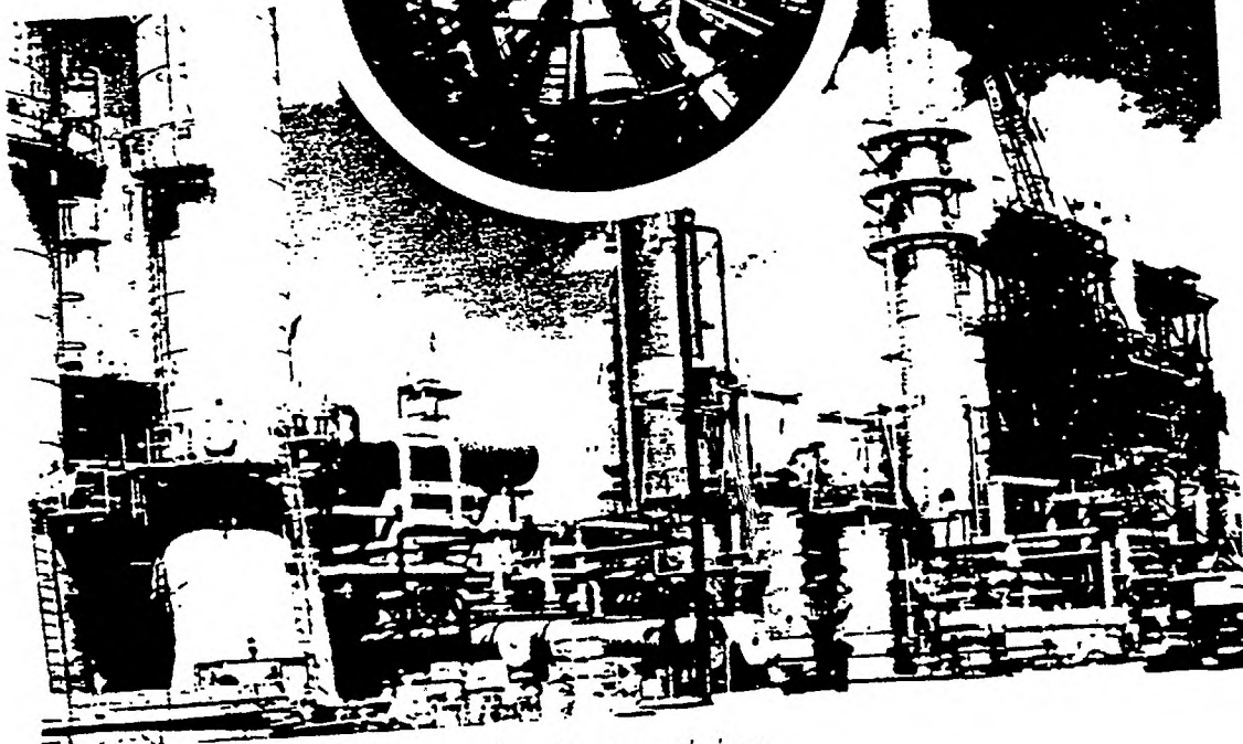
The 500 million pound-per-year Sinclair-Koppers ethylene plant nears completion at Houston, Texas
