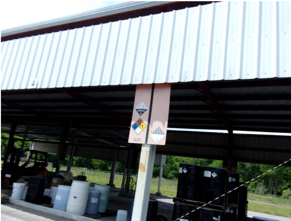
Photo-7 Building 4635-4, Bay 2 Corrosive and Caustic
