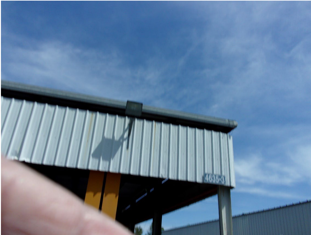
Photo-3 Building 4635-3 Building used for storing hazardous waste and universal waste batteries
