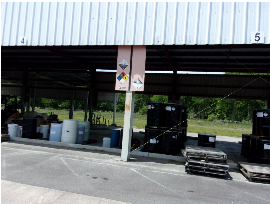
Photo-10 Building 4635-5, Placard labeling as Miscellaneous 9
