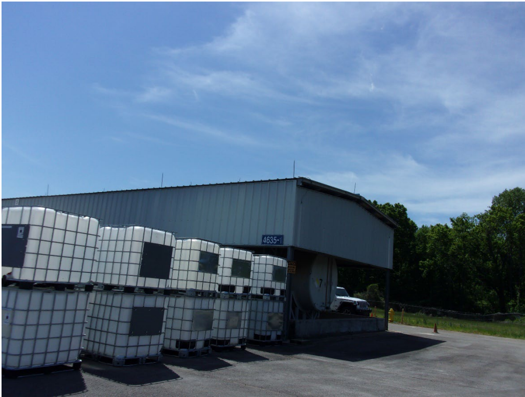
Photo-1 Building 4635-1 storing bulk storage tanks
