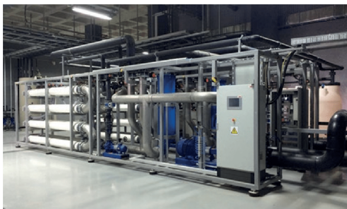
Picture 1. Berghof Membranes B-SMART self-regulating UF Skid
