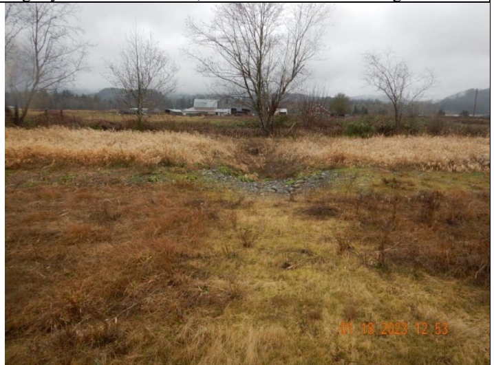
Photo: #26 (DSCN0483.JPG) Description: Facing east, north of Photo 25 photo shows raised dike separating lands leased by Facility from the Drainage District 5 lateral.
