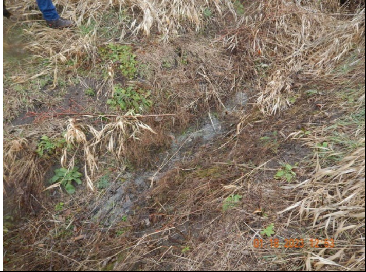
Photo: #27 (DSCN0484.JPG) Description: Surface water flowing north across lands leased by Facility. Water appeared to flow in small channel.
