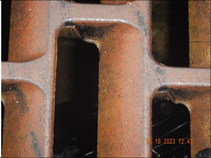
Photo: #23 (DSC0480.JPG) Description: Close-up of catch basin in Photo 22. We noted a pipe leading north from the catch basin back to land owned by the Facility.
