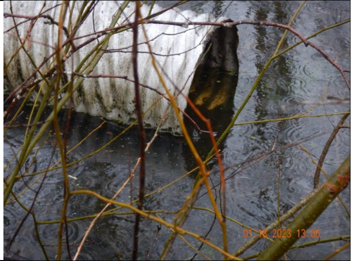
Photo: #40 (DSCN0497.JPG) Description: Close-up of pipe in background of Photo 39. Pond's water level crosses threshold of pipe's lower lip. The pipe appeared to slant up, above stormwater pond level.
