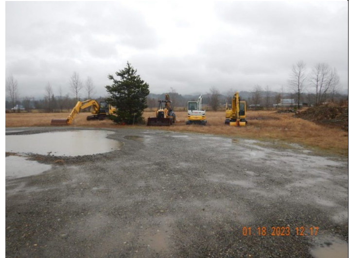
Photo: #04 (DSCN0461.JPG) Description: Facing east, four large earthmoving pieces of equipment stored on-site to test new products manufactured at the Facility.
