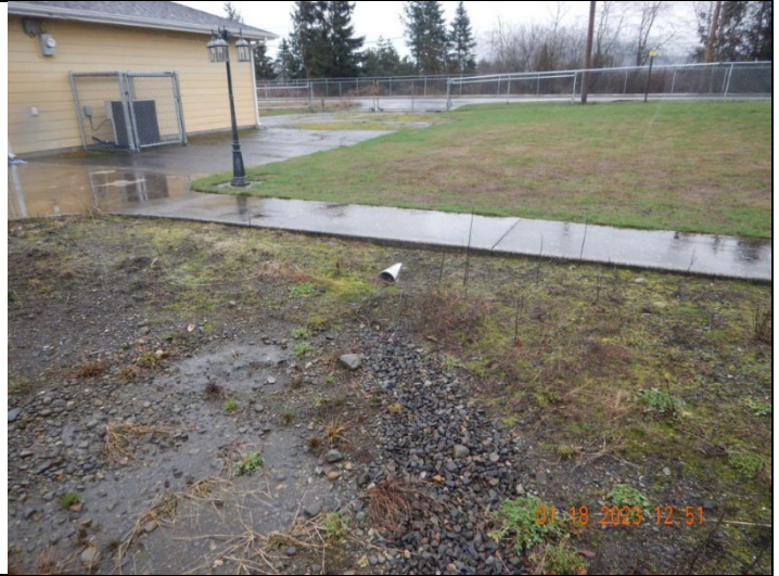
Photo: #24 (DSC0481.JPG) Description: Facing south, with Battersby Avenue in background. Exposed pipe appears to serve as discharge point from the catch basin in Photo 22. Land around pipe appeared slightly lower in elevation, and we saw some standing water.
