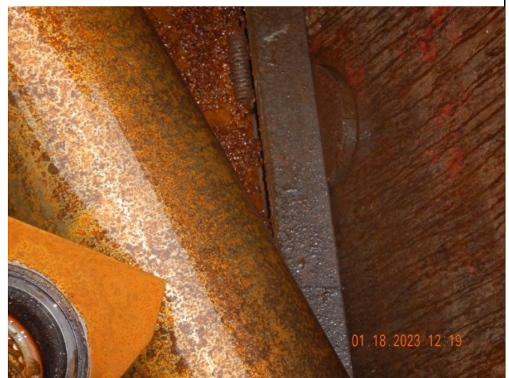
Photo: #06 (DSC0463.JPG) Description: Interior of rightmost dumpster in Photo 5, showing steel scrap and fines, with an open seam at the bottom. Beneath the dumpster appeared rust colored water (pool visible in Photo 5).
