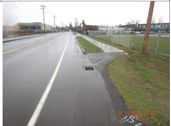
Photo: #22 (DSC0479.JPG) Description: Facing west along Battersby Avenue, looking towards the Facility. Image shows a catch basin along the right of way.
