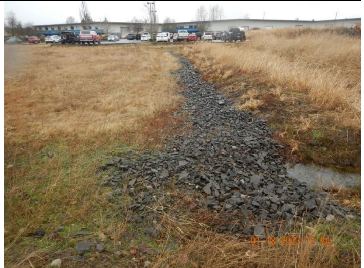
Photo: #30 (DSCN0487.JPG) Description: Facing west towards Facility. Image of channel, and apparent rock dam, carrying surface water generally east and north across lands leased by the Facility.
