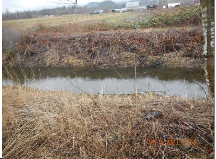
Photo: #28 (DSCN0485.JPG) Description: Facing east, photo shows lateral of Drainage District 5 flowing north from Battersby Avenue.
