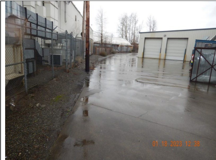
Photo: #19 (DSC0476.JPG) Description: Facing north, turned opposite from vantage in Photo 18, pooling water in previous photos does not appear flowing towards the street.
