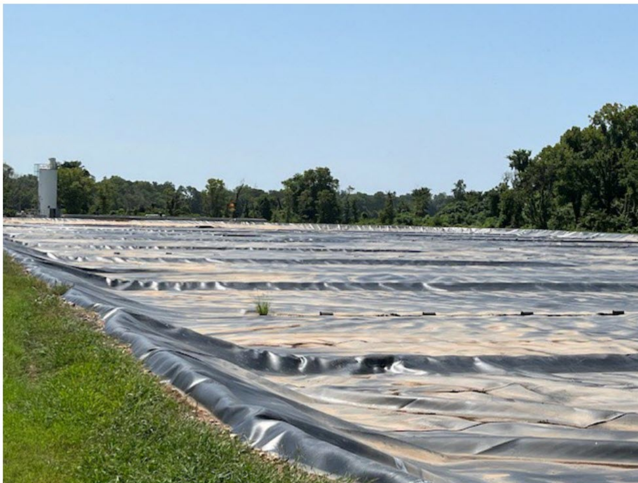
Cover Sedimentation Basin
