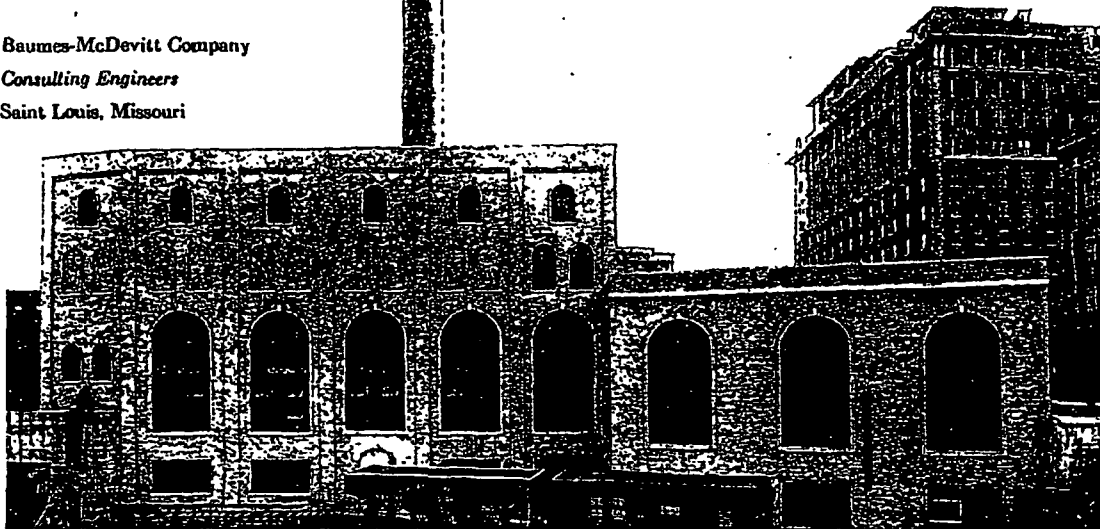
Exterior of Euclid Avenue Power and Service Station of Washington University School of Medicine, St. Louis, Mo. In the rear, the thirteen-story McMillan Hospital, one of a number of hospital buildings covering approximately eight blocks, served by the Station.
