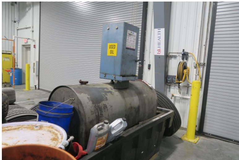
Photo 23: 200-gallon tank in the Grounds/Transportation building labeled "used oil". Located in the Grounds/Transportation Maintenance Area.
