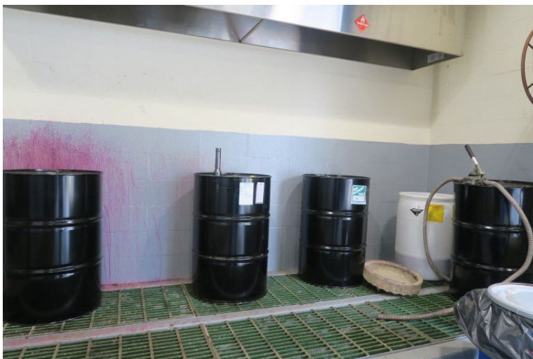
Photo 8: Five containers (four 55-gallon and one 30-gallon drum) on a catch basin in the TSD building. The 30-gallon drum and 55-gallon drum with the hose attachment contained hazardous waste (Carson's solution). The other containers were empty, contained non-hazardous waste, and non-regulated material.
