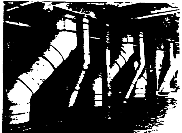
Transite Vents in the World's Largest Distillery Hiram Walker & Sons, Peoria, Ill.
