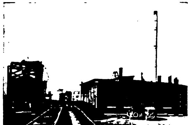
Transite Stack on Roundhouse Power Plant Used for its resistance to corrosive fumes.
