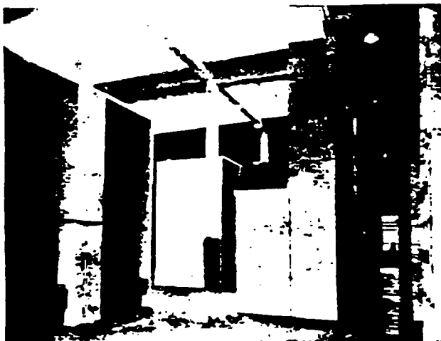
Transite Cell Structure at the Westchester Lighting Company, Port Chester (N. Y.) Plant
