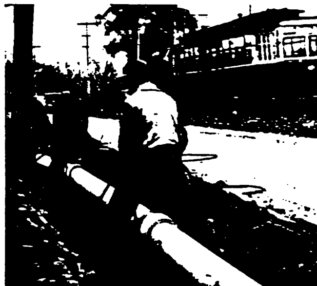
Immunity to Electrolysis Makes Transite Pipe Advisable in Proximity to Electric Railways
