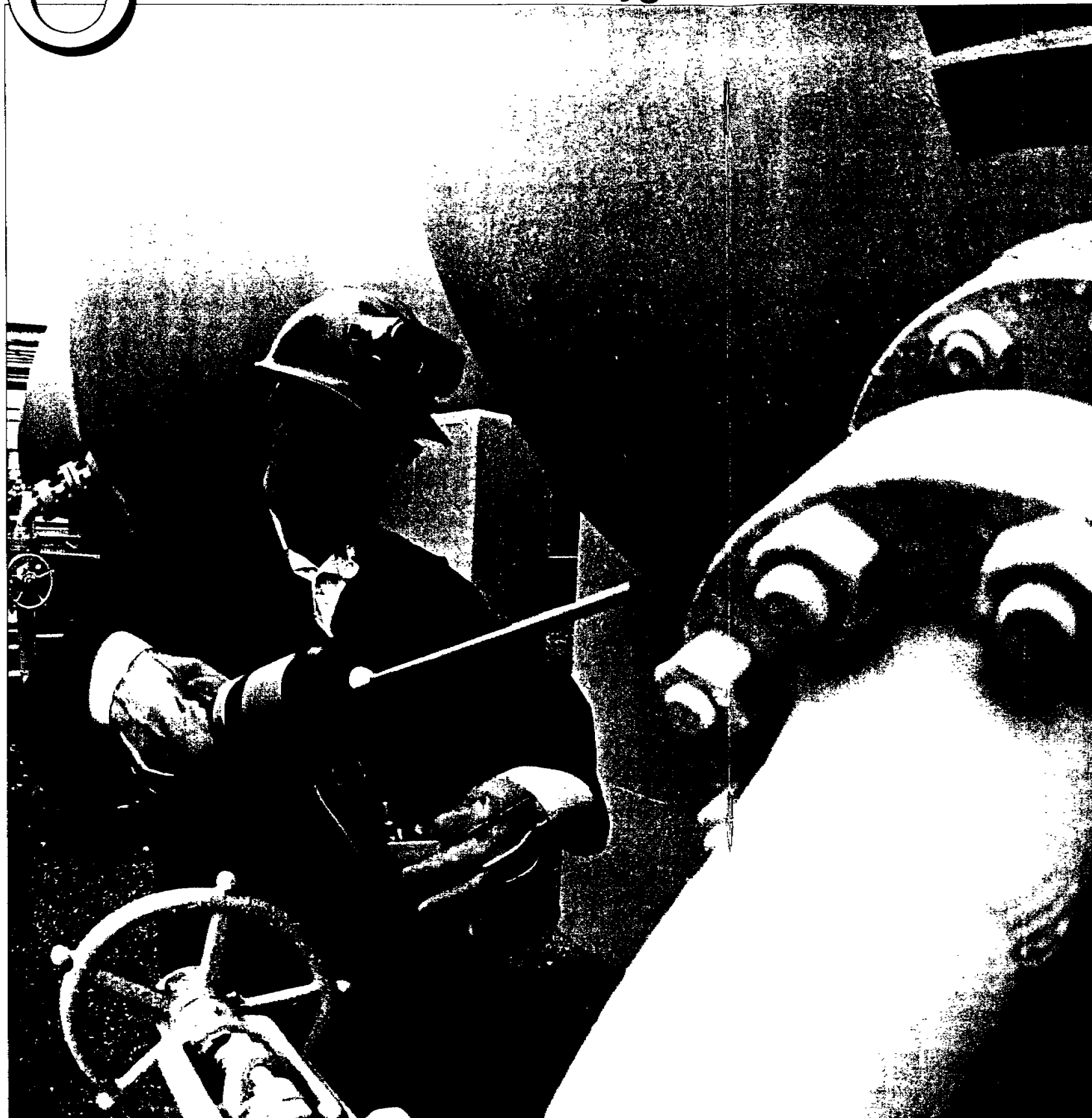
Du Pont industrial hygienist Stephen Dixon checks storage tank for organic vapor leaks, using a photoionization vapor detector.
