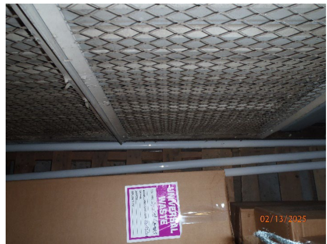
Picture 11 – Building 72 Universal Waste lamps uncontained, not dated, not labeled
