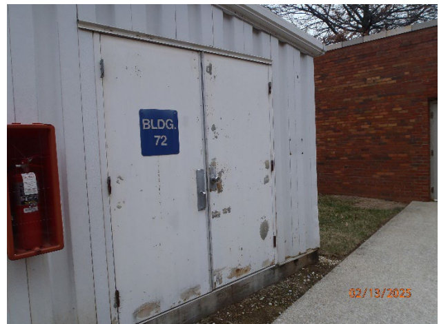
Picture 5 – Building 72 Universal Waste Storage
