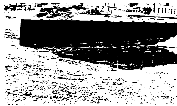
Here are pictures of the newest settling basin, which was recently put into operation. The picture above shows the basin in its final stages of construction in the area just north of the Garage, with the bafflewall to restrict the flow of water complete in the center of the basin. Below is the basin after water had been added. The last traces of any lead in the waste water from the TEL Area is removed in this basin through a special method developed by Research & Development employees.
