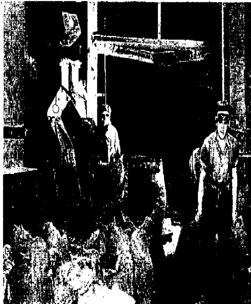
The past, at the beginning of the century, bagging of the fibre and bag handling were entirely manual.
