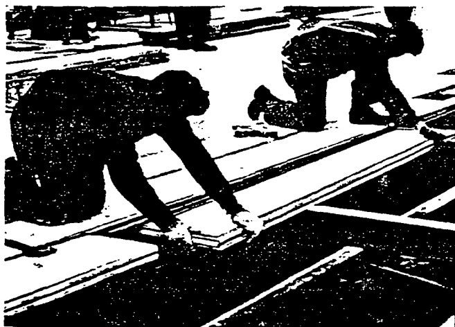
Tongue and groove edges permit USG Gypsum Plank to cantilever. Therefore, ends do not have to meet over supports.
