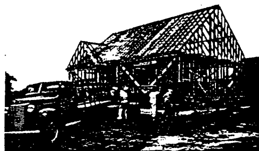
Job started by four mechanics
