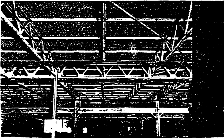
USG Steel Decks look well from within.
