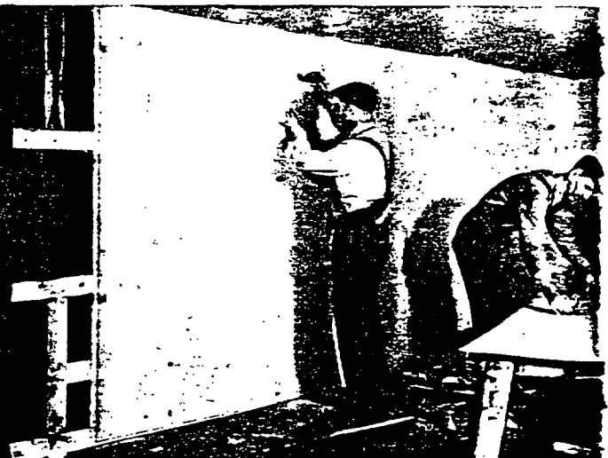
Large sheets permit speedy erection.
