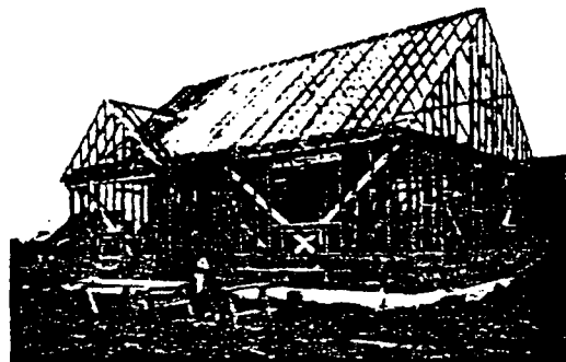
Five rooms, 27' 0" x 36' 0" ready for Gyplap
