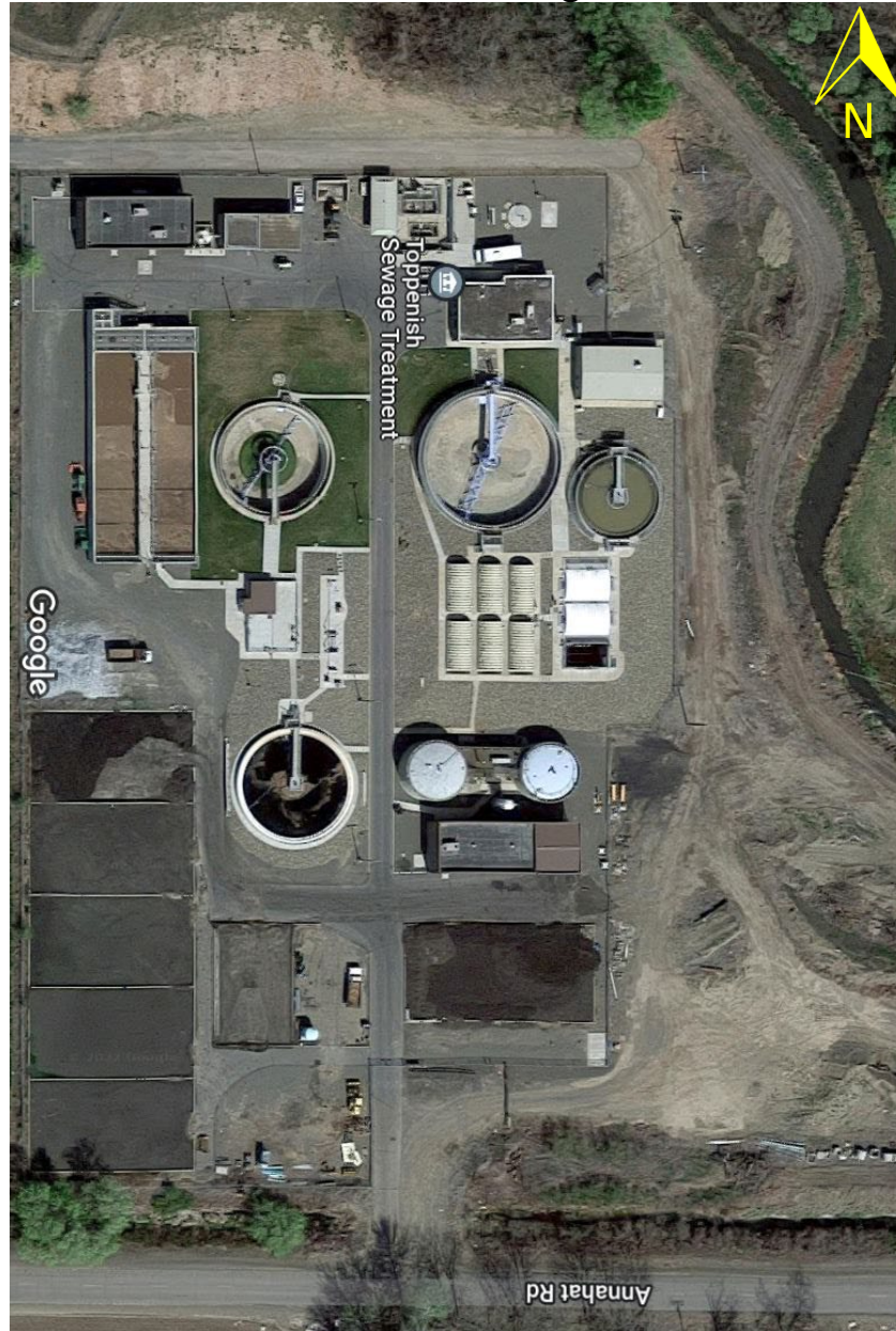
Aerial Site Image
