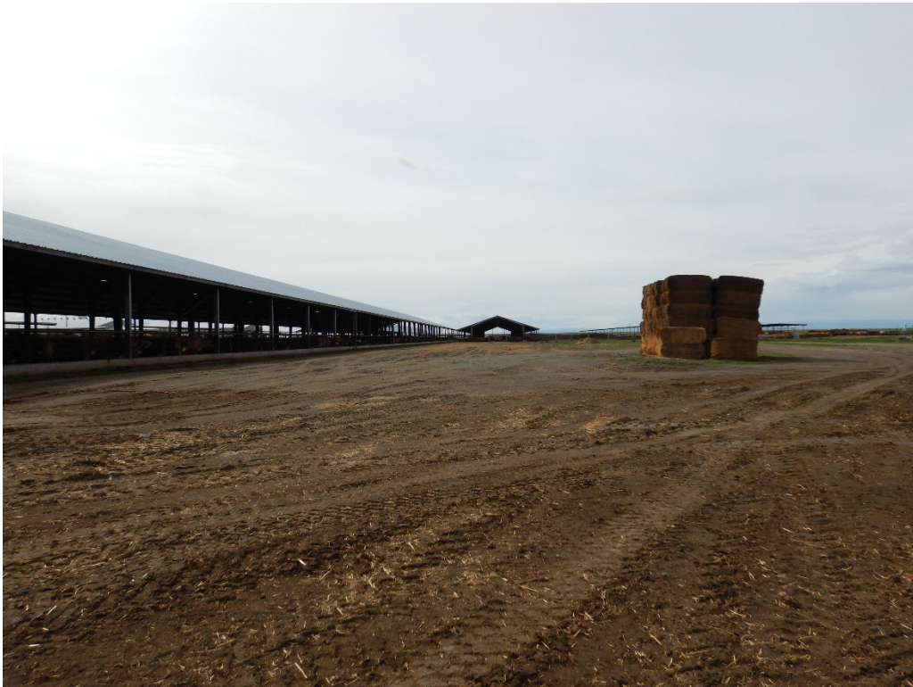
Photograph 13. View looking west from the easternmost end of the production area.
