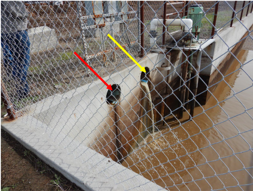
Photograph 6. The north end of the east wall in the Collection Pit. The red arrow indicates the inlet for runoff from building roofs, pen alleys, and feed lanes; the yellow arrow indicates the inlet for wastewater from the milking parlor.
