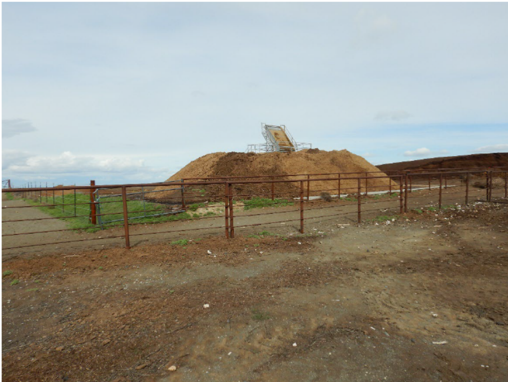
Photograph 7. View looking northeast from the north end of the Collection Pit toward the separator screen and separated solids stockpile.
