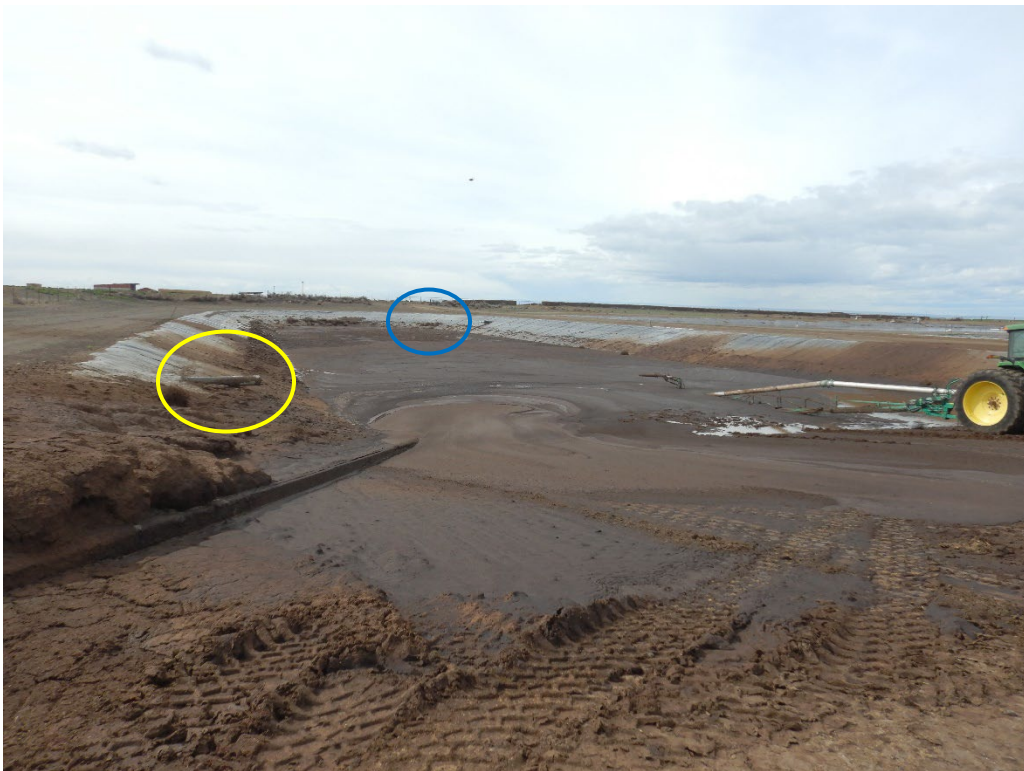
Photograph 2. View looking northwest at the Slurry Lagoon. The pipe in the south berm (yellow circle) is the inlet for silage leachate. The capped pipe in the north berm (blue circle) is the overflow to the Big Lagoon.
