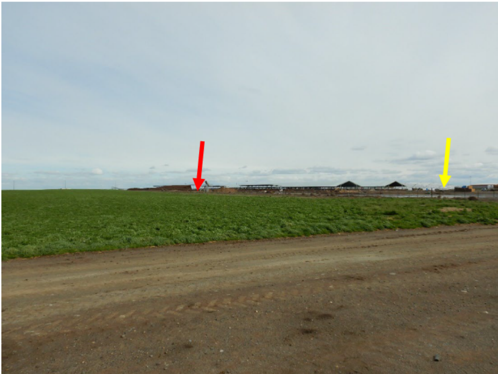
Photograph 29. View looking southwest from the same location as Photographs 27 and 28. The Big Lagoon is visible on the right side of the photo. The red arrow marks the location of the screen separator and separated solids stockpile; the yellow arrow marks the location of the silage bunk.
