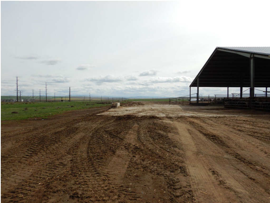
Photograph 14. View looking south, from the same location as Photograph 13, along the southern portion of the east facility boundary.
