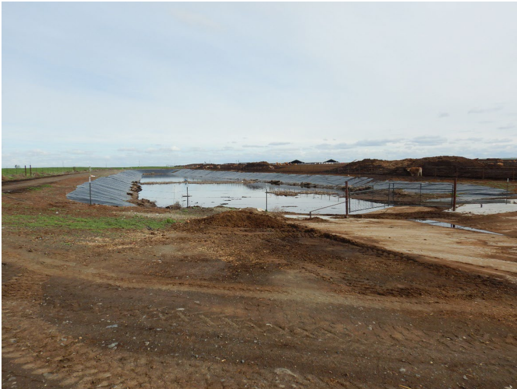
Photograph 26. View looking east, from the same location as Photograph 25, across the Heifer Lagoon.
