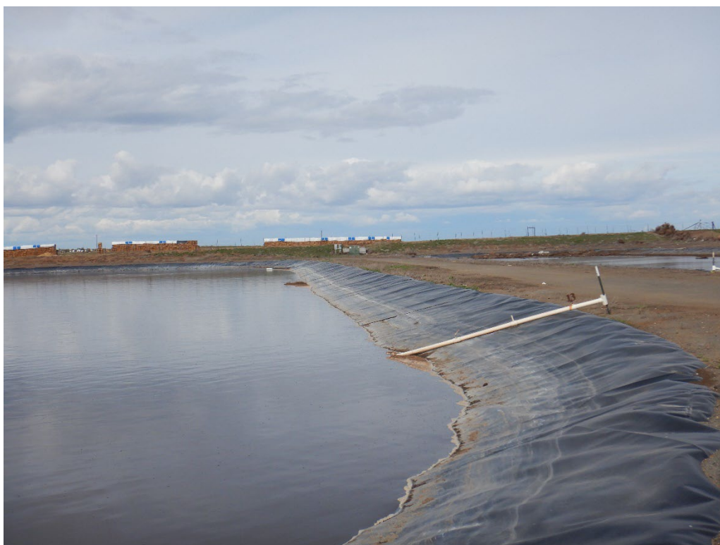
Photograph 9. View looking north at the depth marker located near the southeast corner of the Big Lagoon. The Settling Basin is visible on the right side of the photo (east of the Big Lagoon).
