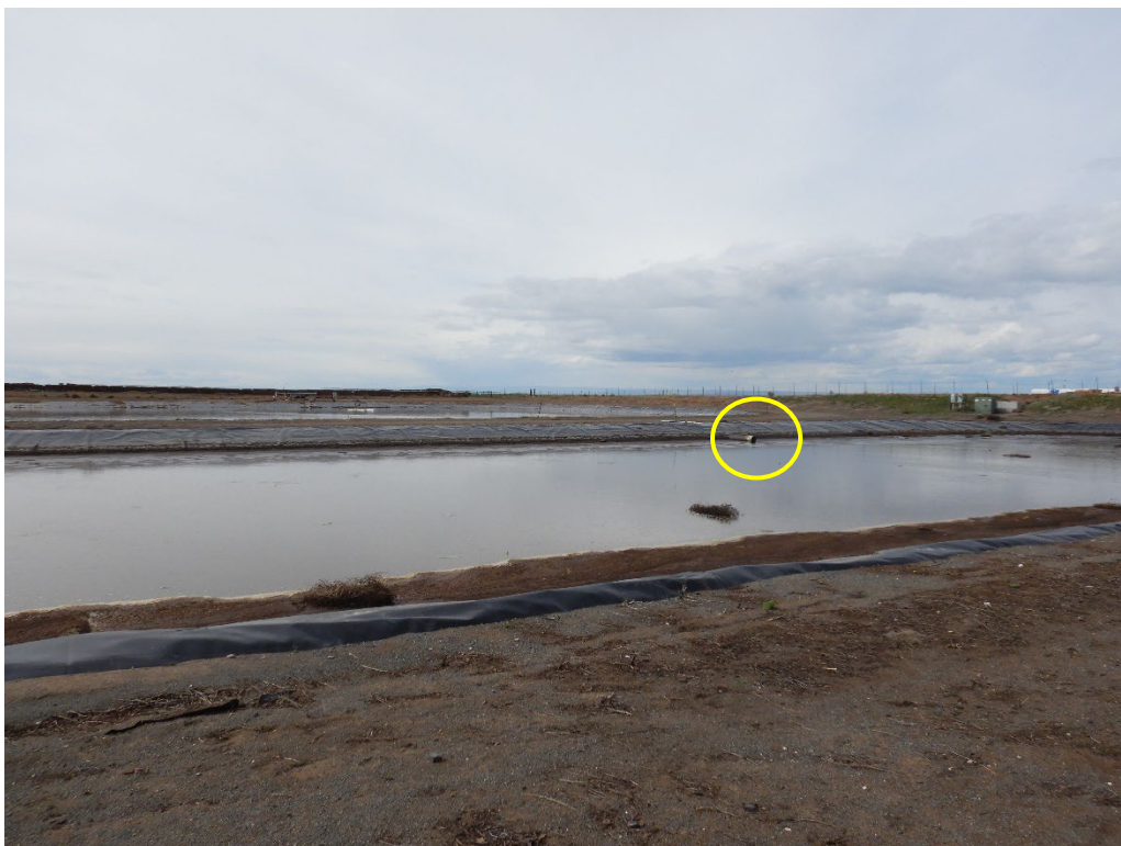
Photograph 8. View looking northwest across the Settling Pond and the overflow pipe (circled) to the Big Lagoon.
