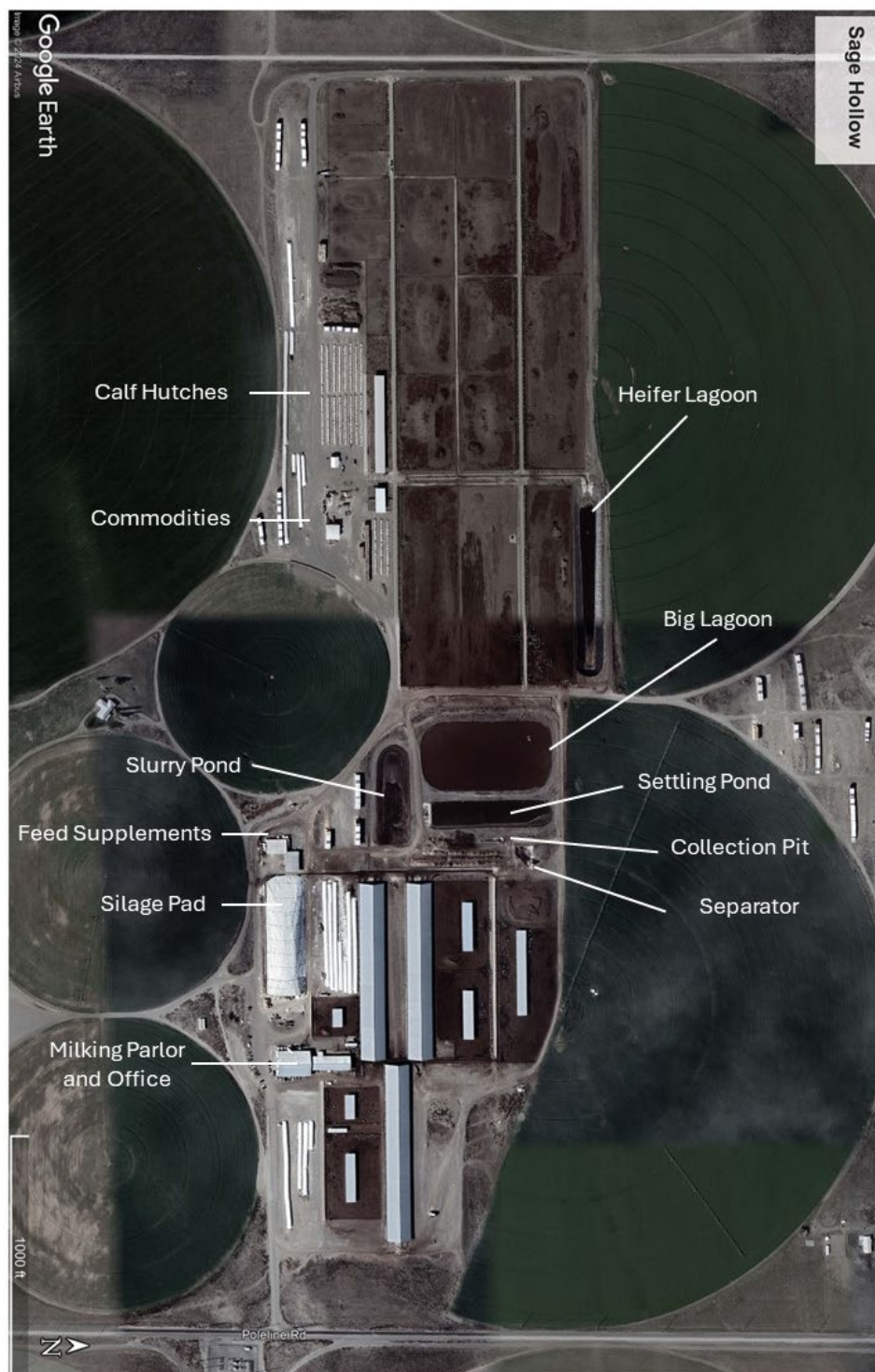
Figure 1. Aerial image of the Sage Hollow Ranch production area.
