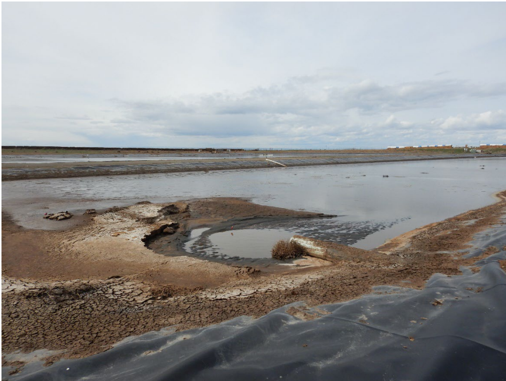
Photograph 4. View looking northwest across the Settling Pond. The pipe in the foreground is the inlet from the manure separator.
