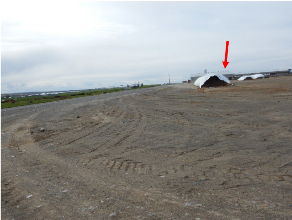
Photograph 16. View looking west, from the same location as Photograph 15, along the southern boundary of the east side of the production area. The arrow indicates the milking barn.
