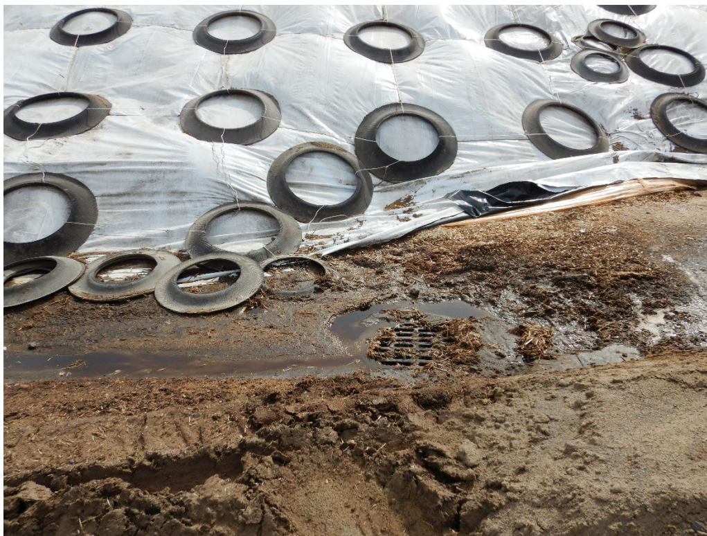
Photograph 1. Silage leachate drains to a manhole (pictured) near the northwest corner of the concrete silage slab; leachate flows through underground piping to the Slurry Lagoon.
