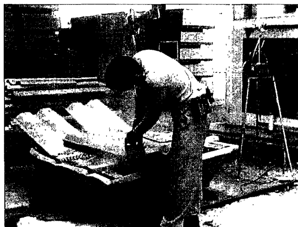
Fig. 4. Motor saw mitering.
