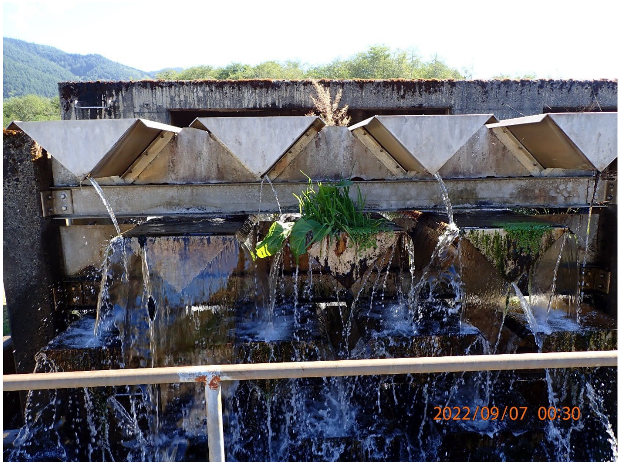
Photo 1/ P9060052 - Degassing area
