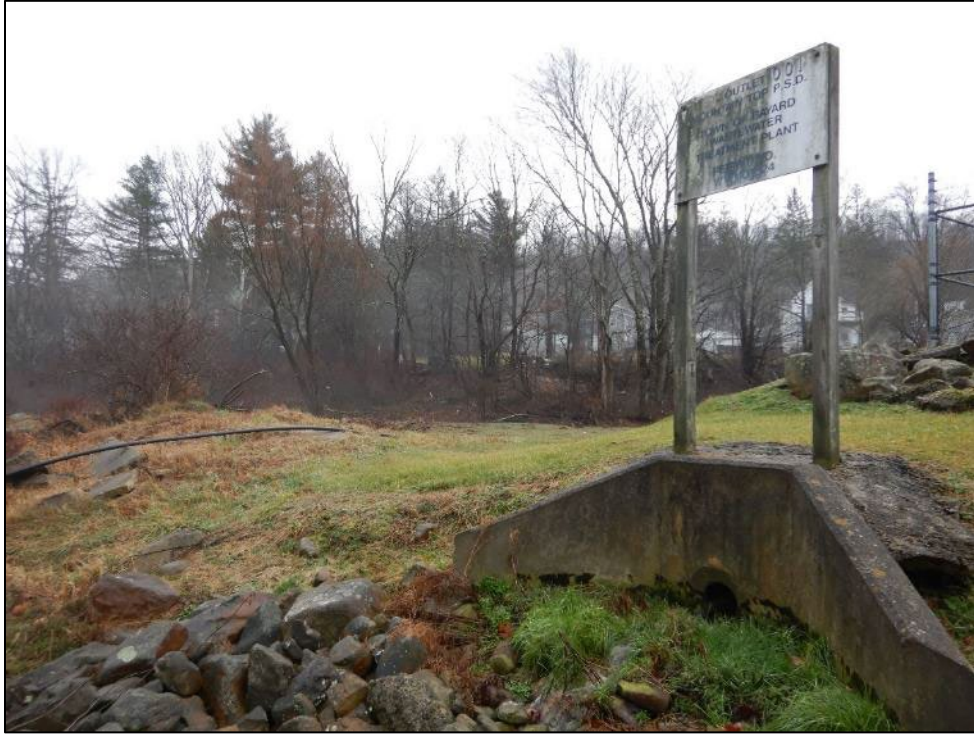
Photograph 37. Bayard WWTP. (DSCN9731) View of Outlet 001 headwall, pipe, and sign.
