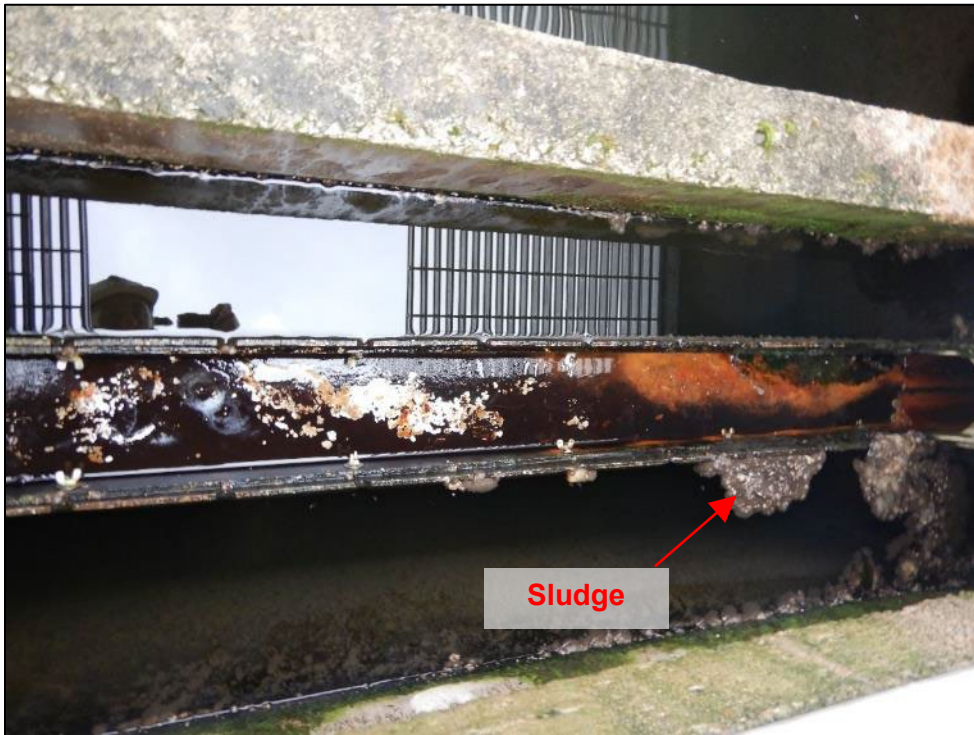
Photograph 28. Bayard WWTP. (DSCN9698) View of the southern clarifier effluent weir. Floating sludge was adjacent to the weir.
