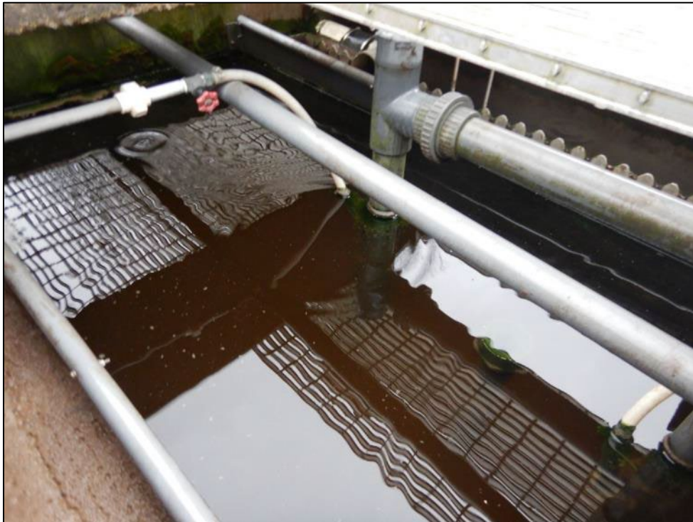
Photograph 6. Gormanian WWTP. (DSCN9615) View inside the clarifier.
