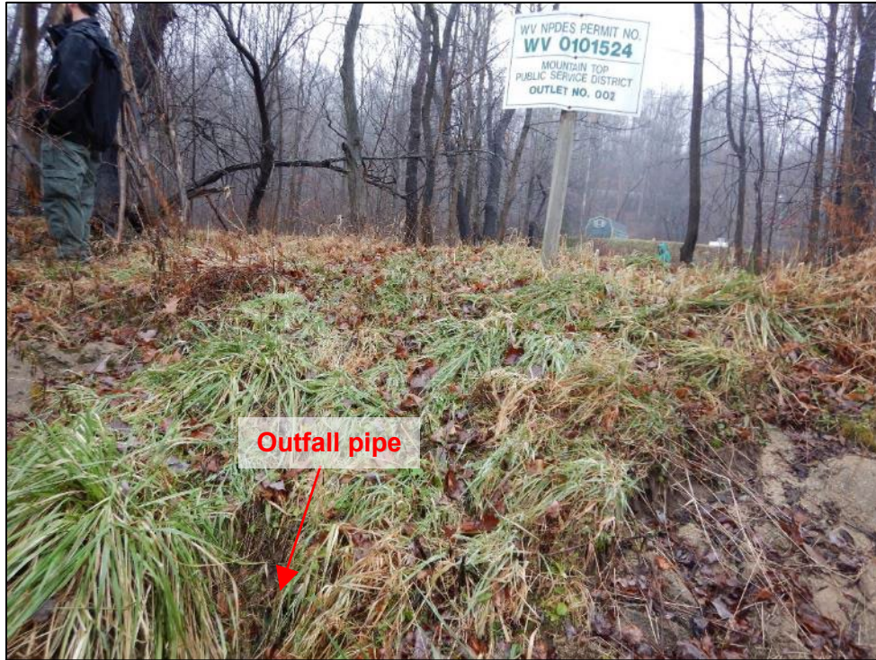
Photograph 13. Gormanian WWTP. (DSCN9641) View of Outlet 002 and sign. The arrow callout is pointing to the general position of the outfall pipe as it is obscured from view by vegetation (refer to Photograph 14).
