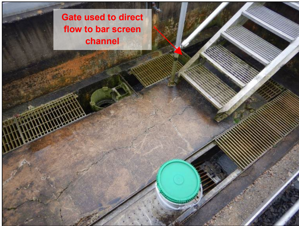
Photograph 19. Bayard WWTP. (DSCN9673) View of the influent channels. There are two channels, one that had been equipped with a grinder that had been removed from service. The other is equipped with a manual bar screen. At the time of the inspection, influent flow was directed to the manual bar screen channel.
