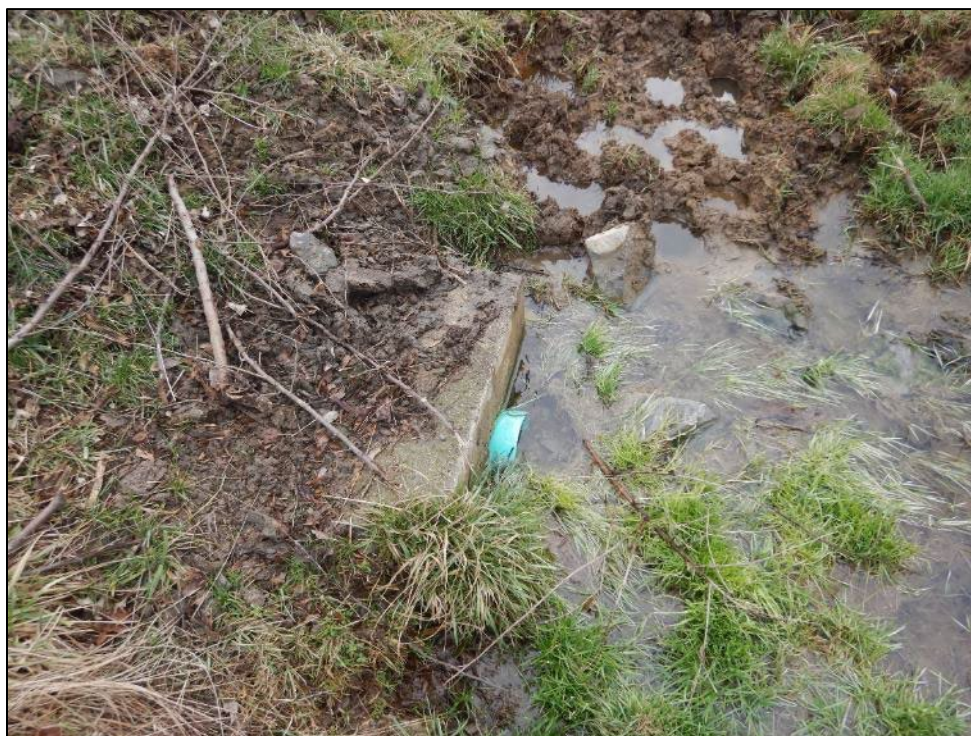
Photograph 64. Elk Garden WWTP. (DSCN0023) View of Outlet 003 pipe.
