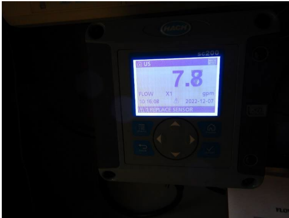
Photograph 12. Gormanian WWTP. (DSCN9629) View of the effluent flow meter display, which showed a flow rate of 7.7/7.8 gpm at the time of the inspection.
