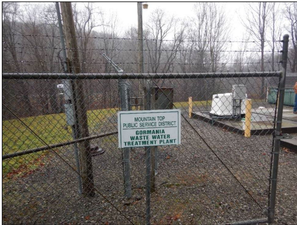
Photograph 1. Gormanian WWTP. (DSCN9604) View of the Gormanian WWTP sign on the entrance gate. The WWTP was surrounded by a chain-link fence with barbed wire. The fence was in good condition at the time of the inspection.
