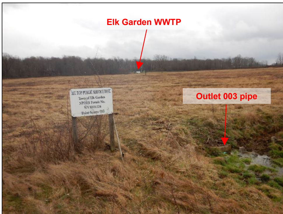
Photograph 63. Elk Garden WWTP. (DSCN0021) View of Outlet 003 pipe and sign. Outlet 003 is located in a cow pasture and approximately 930 feet from the chlorination/dechlorination building.
