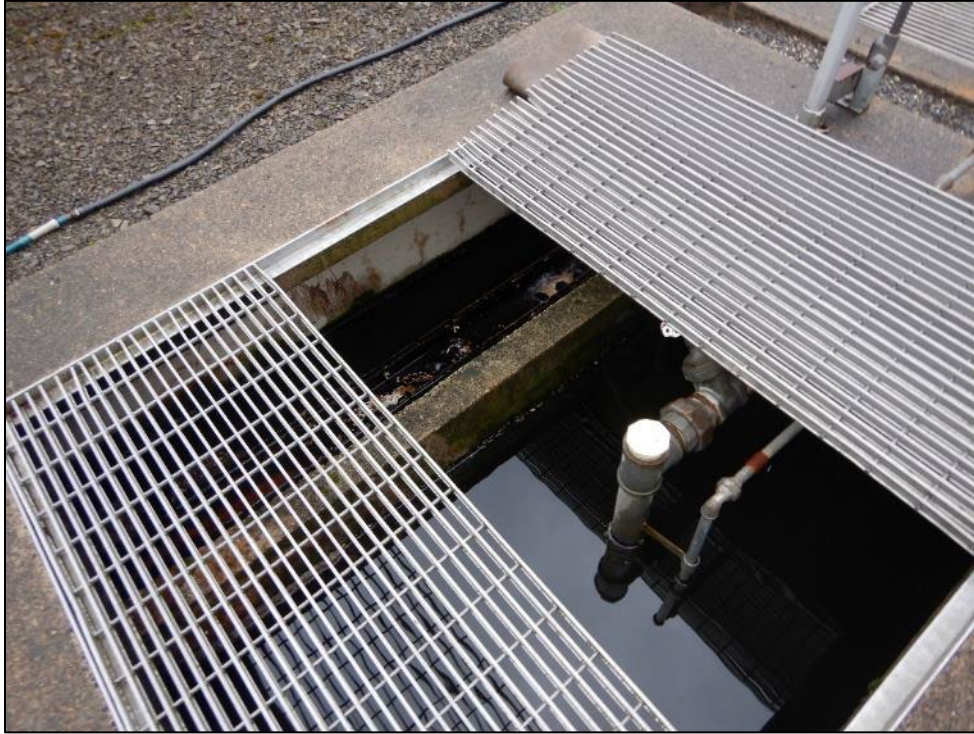
Photograph 27. Bayard WWTP. (DSCN9697) View of the southern clarifier.
