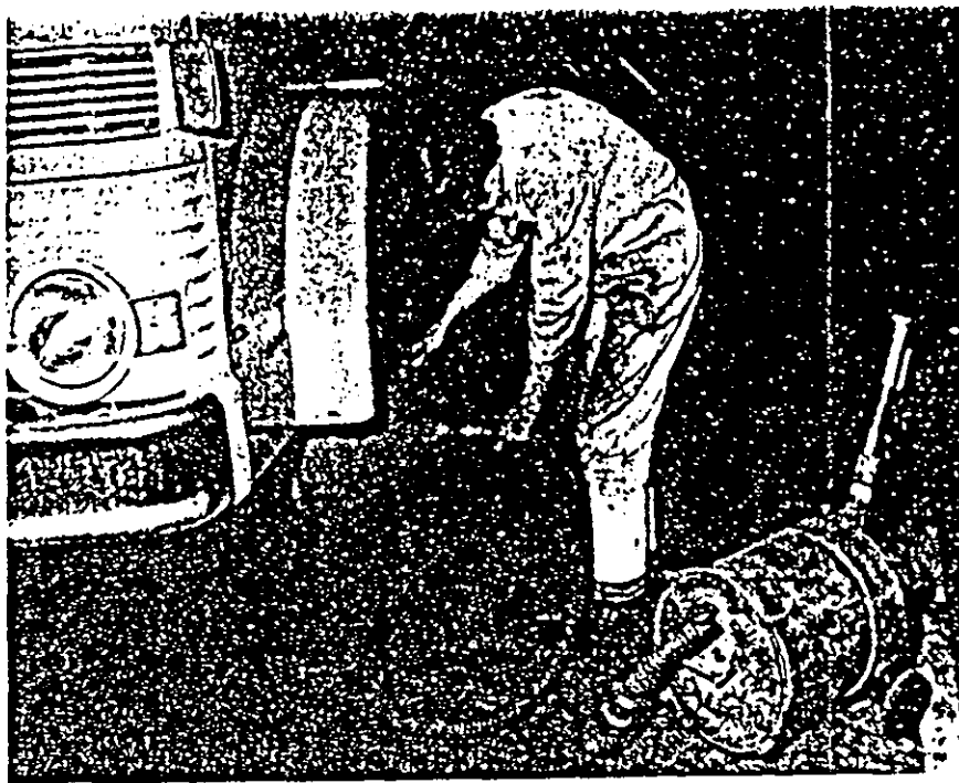
FIG. 1. Funnel method of dust control.
