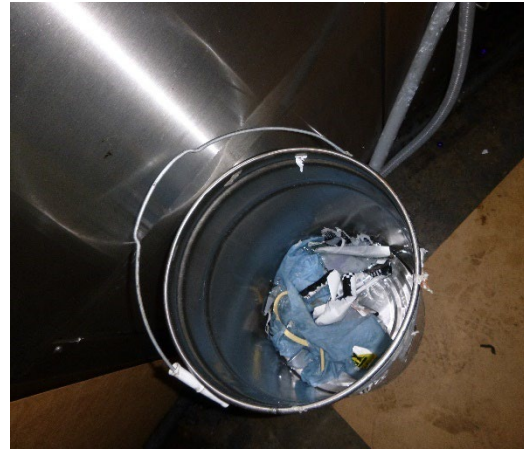
Photograph 26: blue shop towels disposed of - P1030633.JPG
