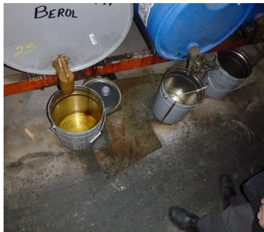
Photograph 22: catch buckets - P1030629.JPG
