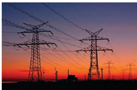
Reducing climate impact of the energy sector
