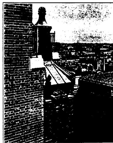
Hard lead spandrel and finial
