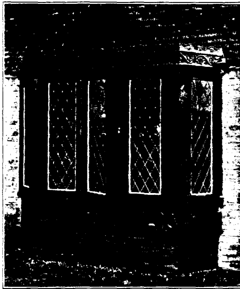
WURTS BROS. Leaded window with ornamental lead frieze and lead flashing on Mr. Heine's small office building
