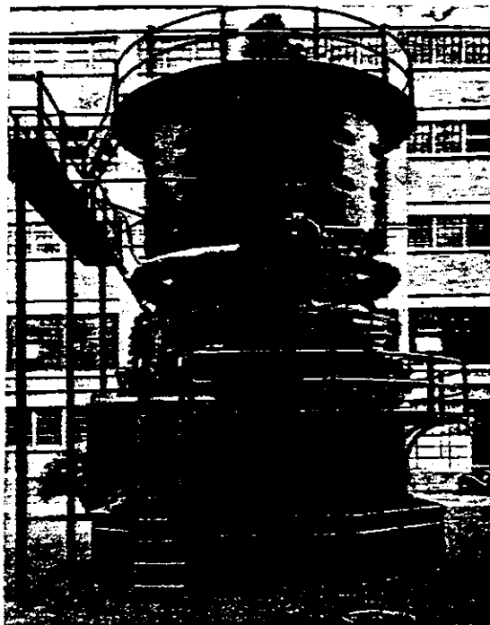
Fig. 3. The first 5000-kw steam turbine generating unit installed at the old First Street Station in Chicago in 1902. This was the largest unit ever built at that time, and First Station was the first all steam turbine electric generating plant built in this country. Curiously enough, First Station today has installed in it the largest single-shaft steam turbine unit ever built. This unit is shown in Fig. 4.
