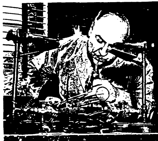
Vince cuts a large diameter glass tubing by means of a hot wire followed by cold water.
