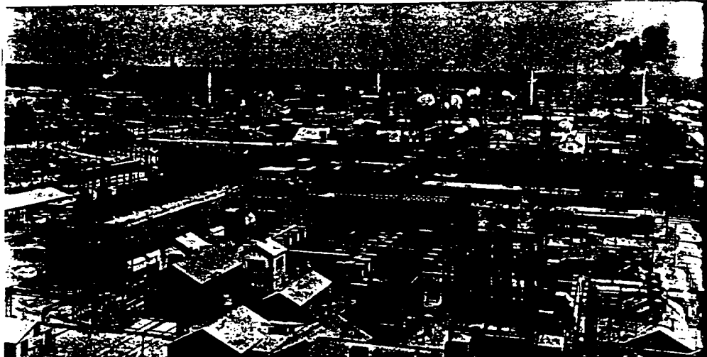
A third wing was added to the sodium area, above, to provide the plant's requirements for sodium & chlorine. They are produced by electrolysis of molten salt heated to high temperatures in an improved type of sodium cell.
