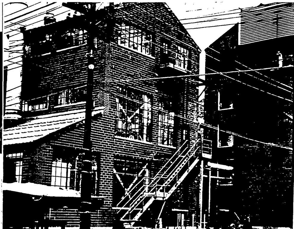
Our sixth TEL building, right, and its adjoining wash house will be among the major new units completed at the Baton Rouge plant this month. Here workmen are painting a ventilating stack
