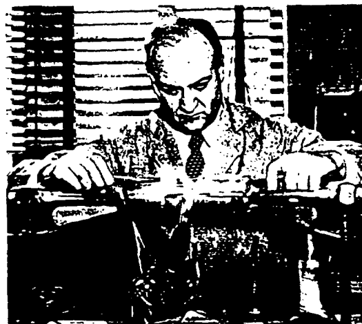
A low-temperature condensing trap in process of construction. Here the bottom is closed.
