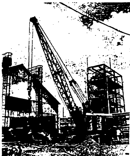
A third wing was added to the sodium area, above, to provide the plant's requirements for sodium & chlorine. They are produced by electrolysis of molten salt heated to high temperatures in an improved type of sodium cell.
