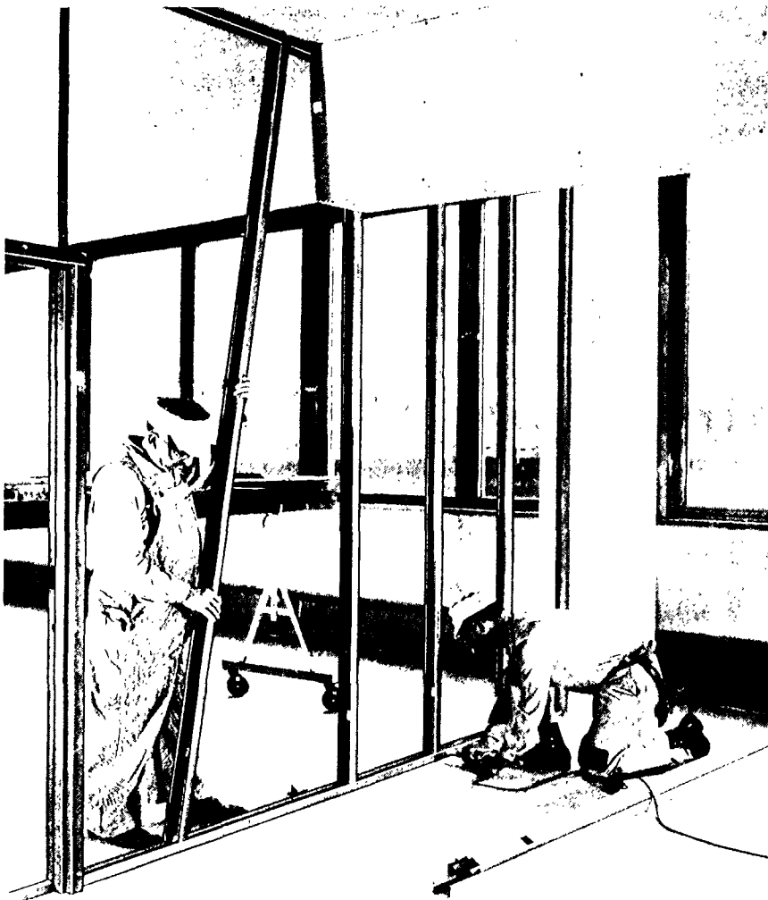
Fig. 21 Metal studs go up quickly in this office building.
