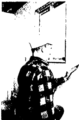
Fig. 66 Smooth, flat and carefully butted joints in vinyl coverings on wallboard are difficult to see.
