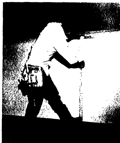
Fig. 16 Gypsumboard can be cut by scoring and breaking. Here, a drywall applicator scores a measured length using a straightedge as a guide.
