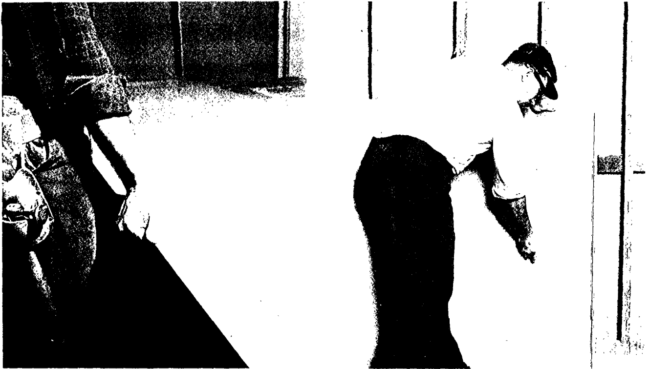
Fig. 17 Completes the break by snapping the gypsumboard away from the scored surface (left) and running a knife through the uncut paper (right). Usually, gypsumboard will be snapped as well as cut while standing as shown at the right.
