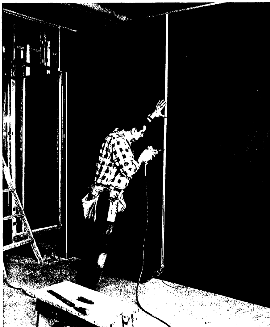
Fig. 54 Some gypsumboard joints, such as these on predecorated panels, are decorated with metal battens. Vinyl inserts are used to hide fasteners.
