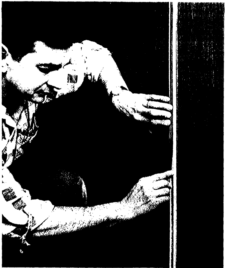
Fig. 64 Screws holding predecorated wallboard are concealed with vinyl strips in battens which cover joints.
