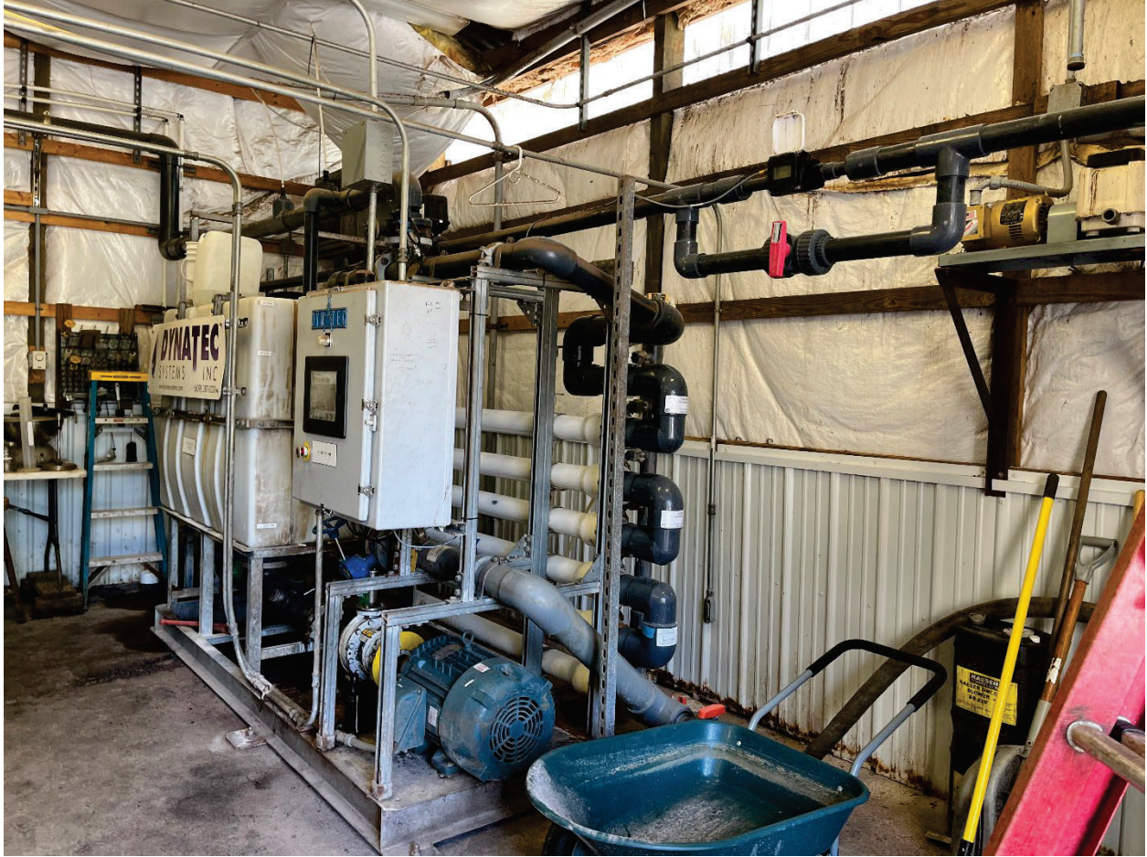
Photograph 5: The effluent then flows in sequence through an Ultra Filter Membrane filter system.
