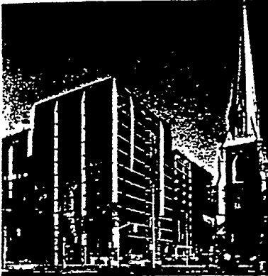
Crane plumbing fixtures were chosen for the new Bank of Canada complex in Ottawa.
