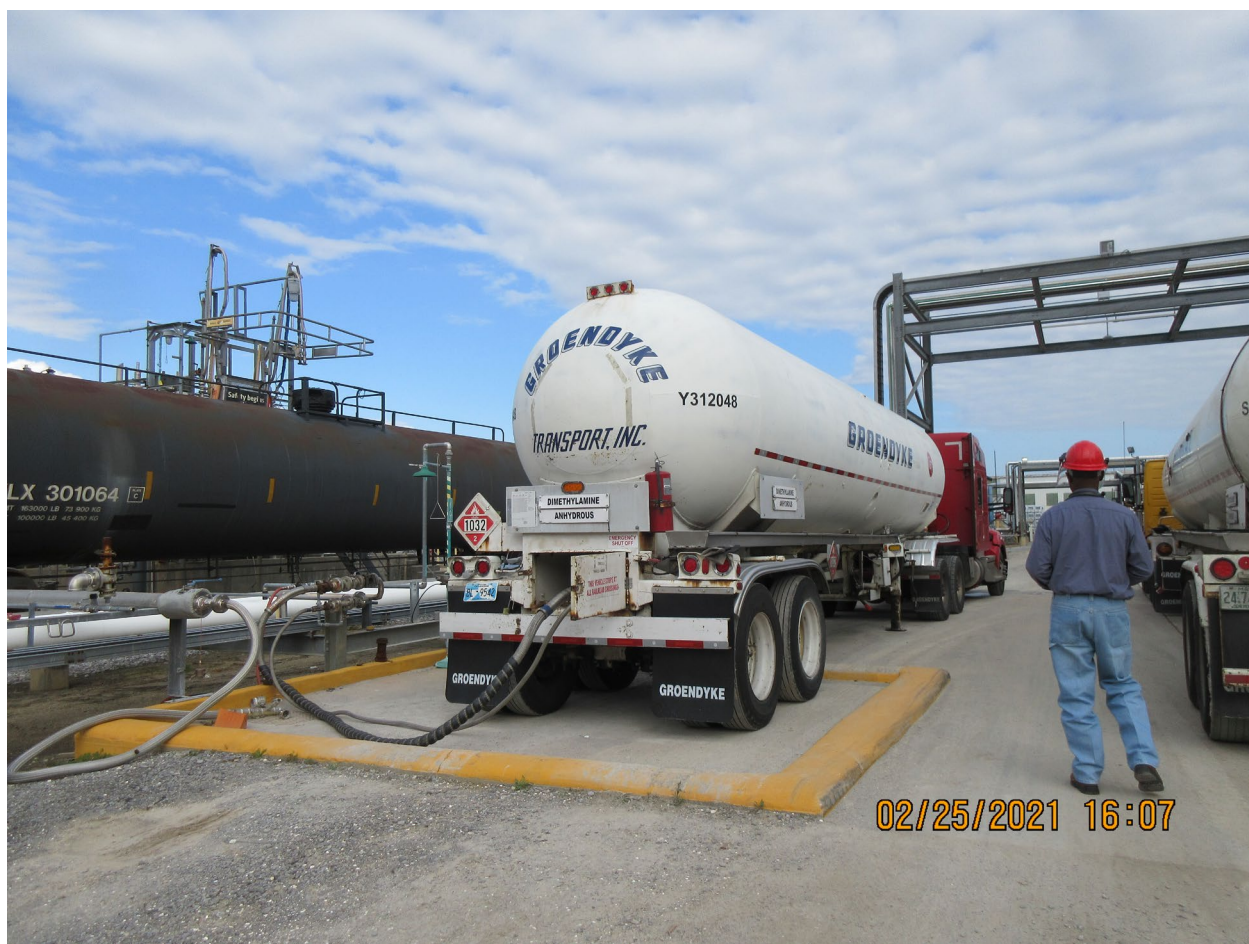
Photo 7 – Tanker Truck Loading Area #6
