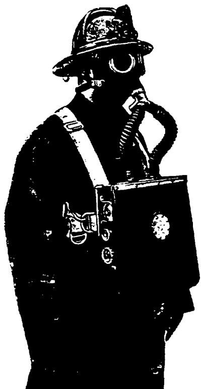
FIG. 2 HALF-HOUR OXYGEN-BREATHING APPARATUS—APPROVED BY THE BUREAU OF MINES (2)
