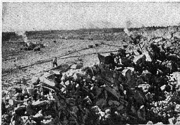
A close-up of the rock pile after a blast. The driller, shown at left center, is preparing for a secondary shot
