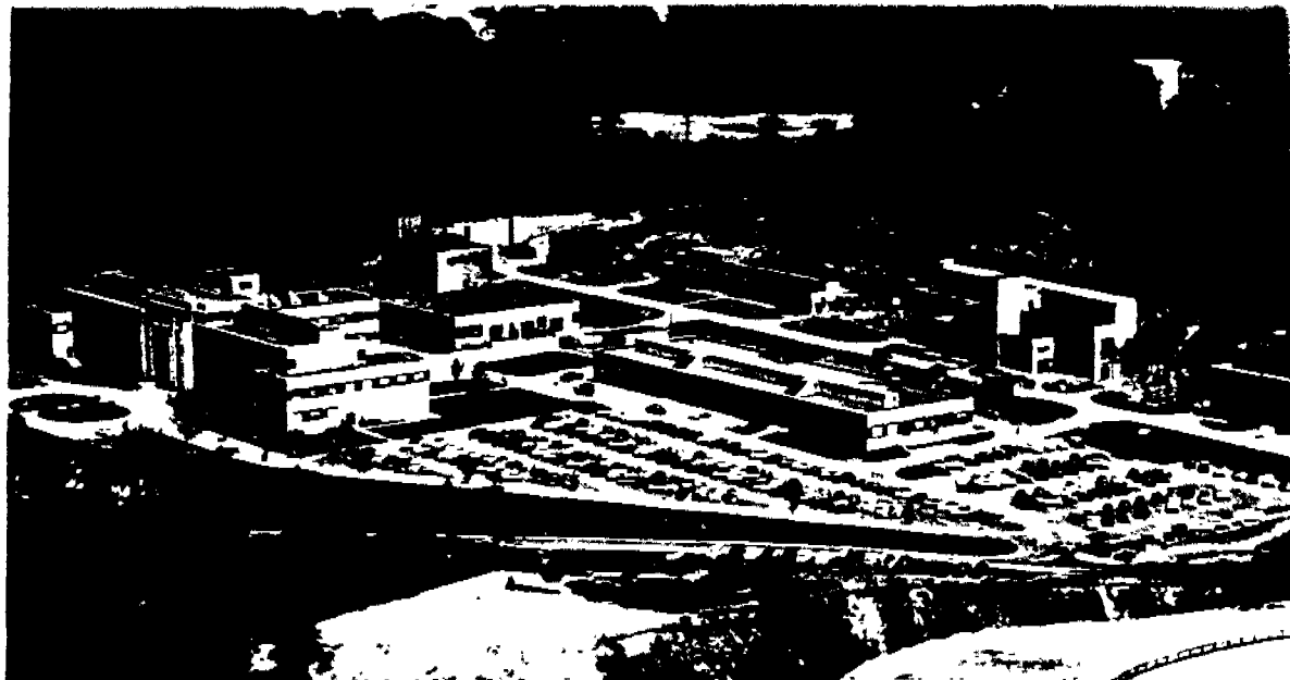
CARBIDE's Research and Development Center at South Charleston, West Virginia—the birthplace of many new chemicals—was first completed in 1949. A new Development and Engineering Center is being built adjacent to present extensive research facilities.
