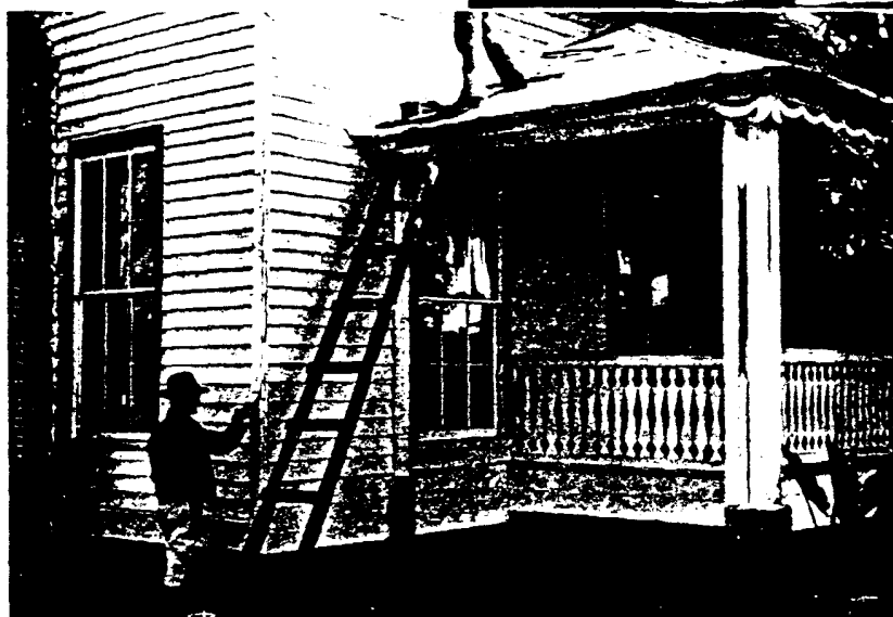
Lower Left—Applying the second coat to one of the houses
