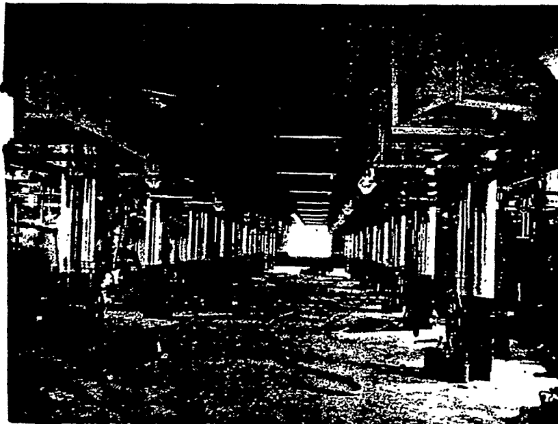
One of the first manufacturing plants when under construction at Deepwater, N. J. in 1926. This building is no longer used.
