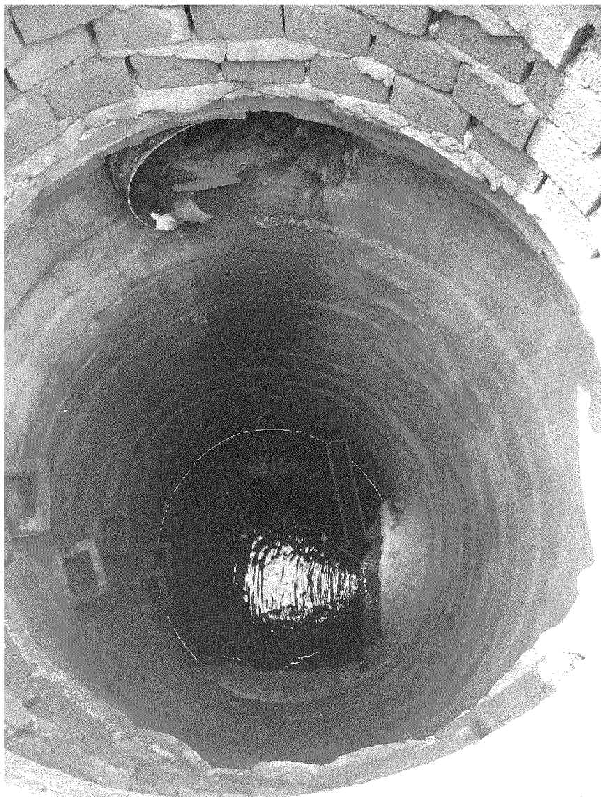
MH-4564950: RIDOT access manhole near the wastewater treatment plant on Ocean Road. Sample collection point indicated by a red arrow.
