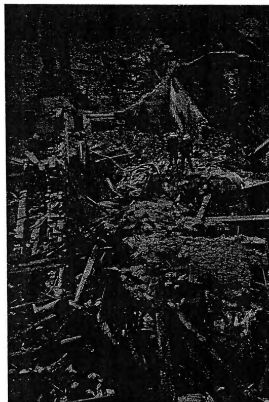
Fig. 8. Wreck of a factory following on the ignition of a starch dust cloud. Eighteen workers were killed and many injured
