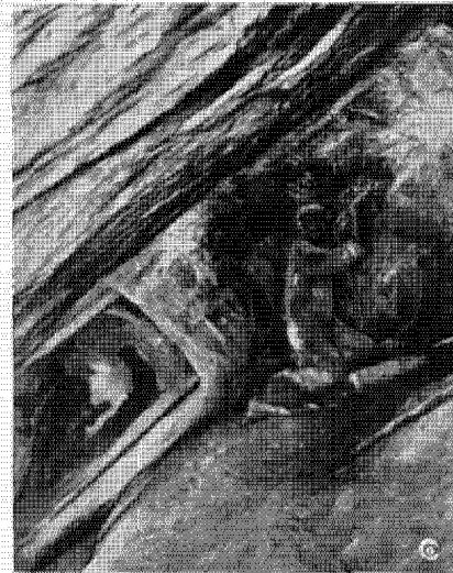
Miners at work in a gold-bearing vein. Notice the pitch of the reef
