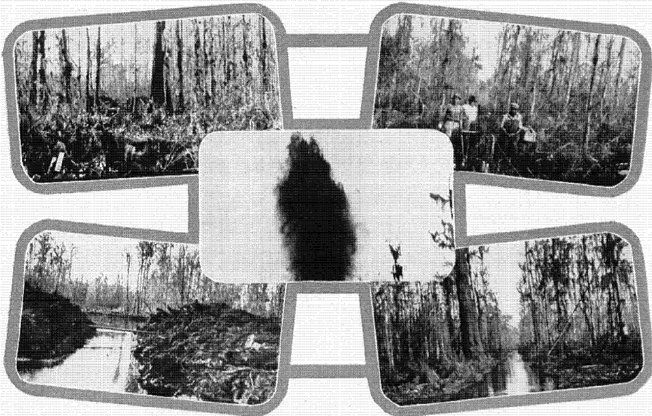
Top, left—Where the right of way for the ditch was cleared. Top, right—Loading holes for the shot. Center—The blast rose above the treetops. Below, left—The cut through the spoil bank. Right—A section of the completed ditch. Note the Spanish moss on the trees
