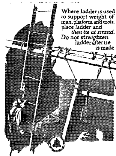
Figure 4. A safe convenient means of lashing a splicer's ladder to the suspension stand.
