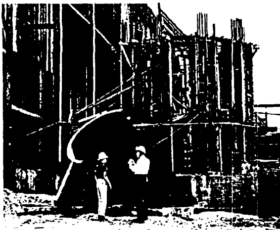
Construction of additional productive capacity at the Adrian Joyce Works is now under way to meet the increasing demand for titanium dioxide pigments.
