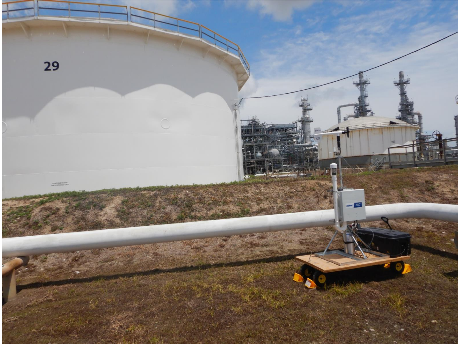
Photo 1161: EPA 1B location near Tank 29, facing N 5/2/23 12:37 DSCN1161.jpg
