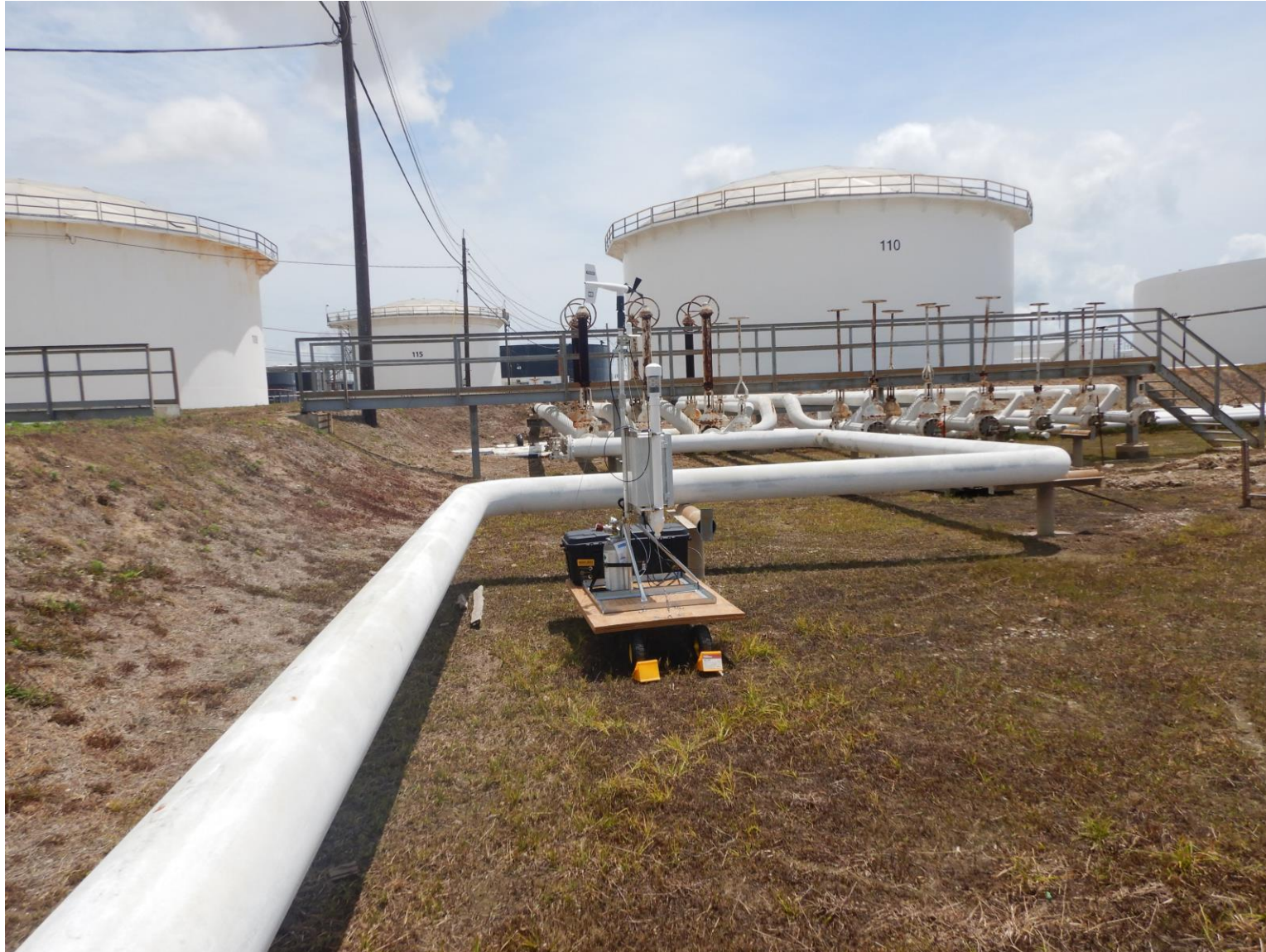
Photo 1162: EPA 1B Location facing E - 5/2/23 12:37 DSCN1162.jpg
