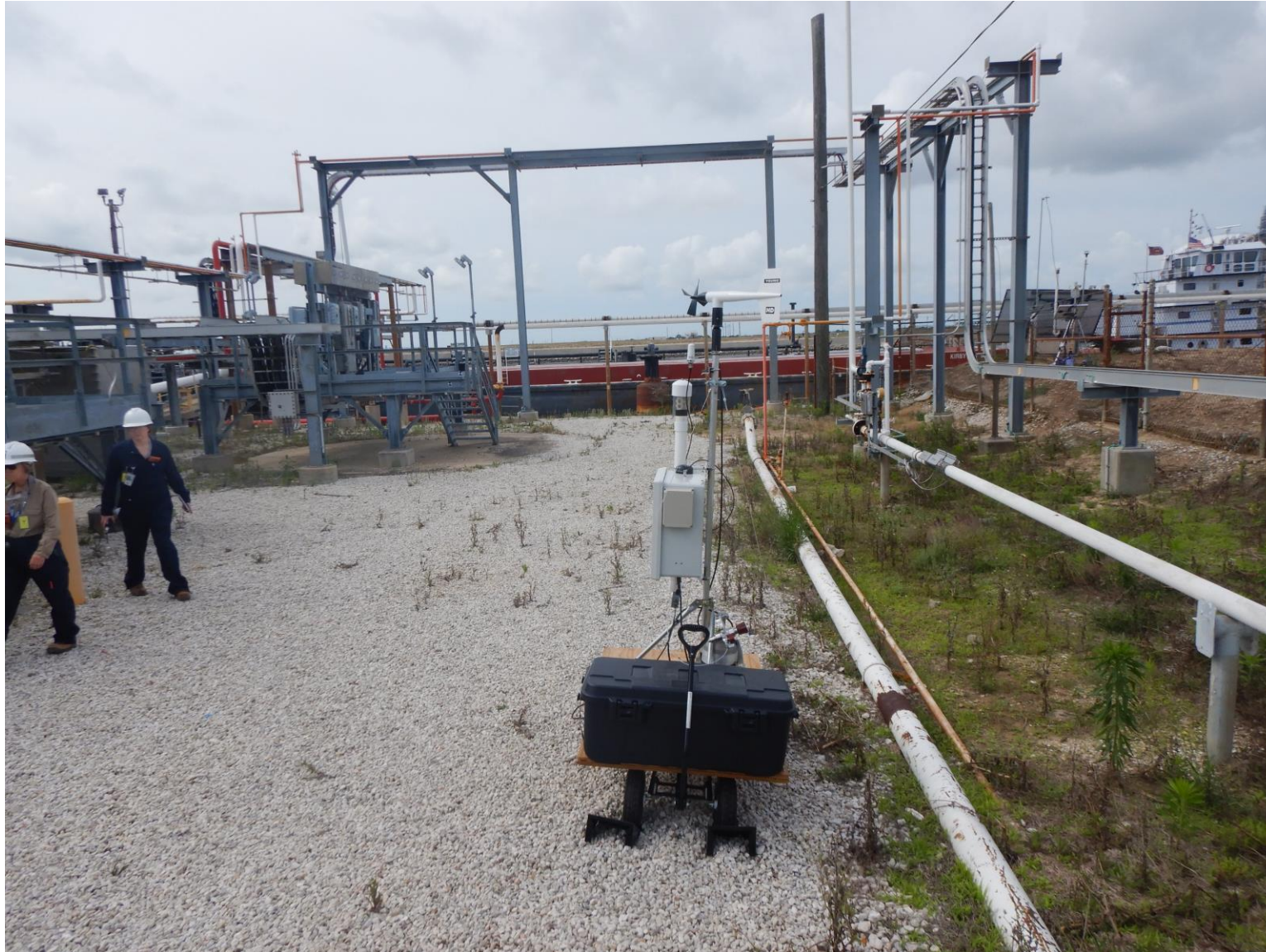
Photo 1159: EPA 2A Location near Dock 54 facing S - 5/2/23 10:10 DSCN1159
