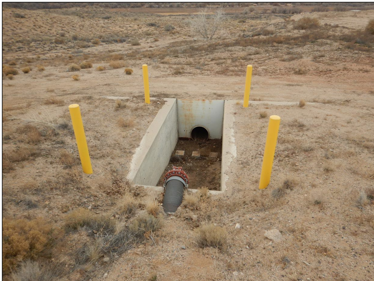
Photograph 18. W0002 Pump-to-Waste Discharge Pipe View of the pump-to-waste discharge pipe northwest of the W0002 building. The pipe discharged into a concrete walled basin which was dry.
