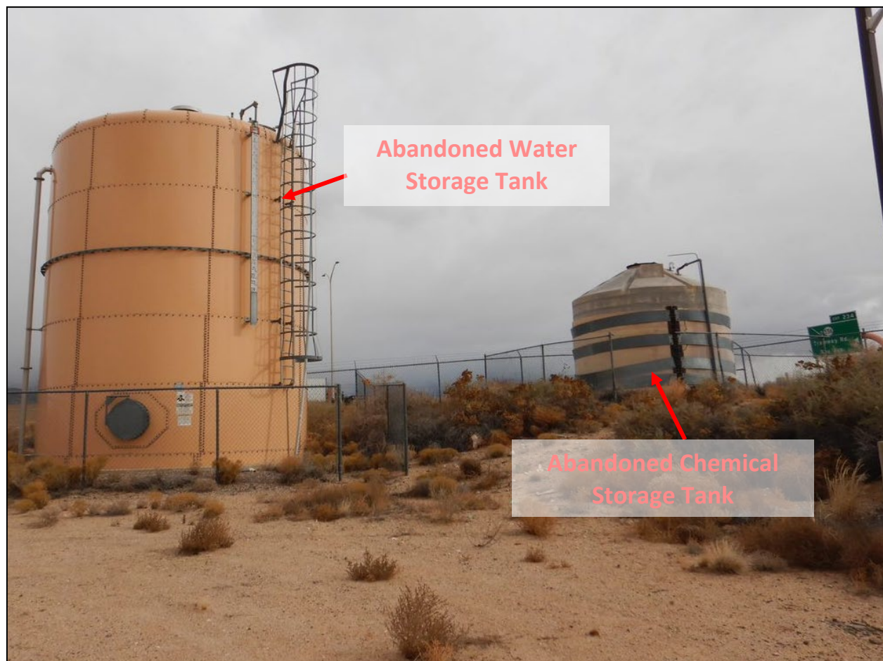
Photograph 1. Abandoned Water Storage and Chemical Storage Tanks View of the abandoned water storage tank and chemical storage tank which were used to support the old casino that was located on the western side Interstate 25 from the new casino, and adjacent to the site of the old police station. The EPA Inspection Team could not locate the abandoned well associated with assets, but they received a well plugging record that documented removing the asset connections to the distribution system.
