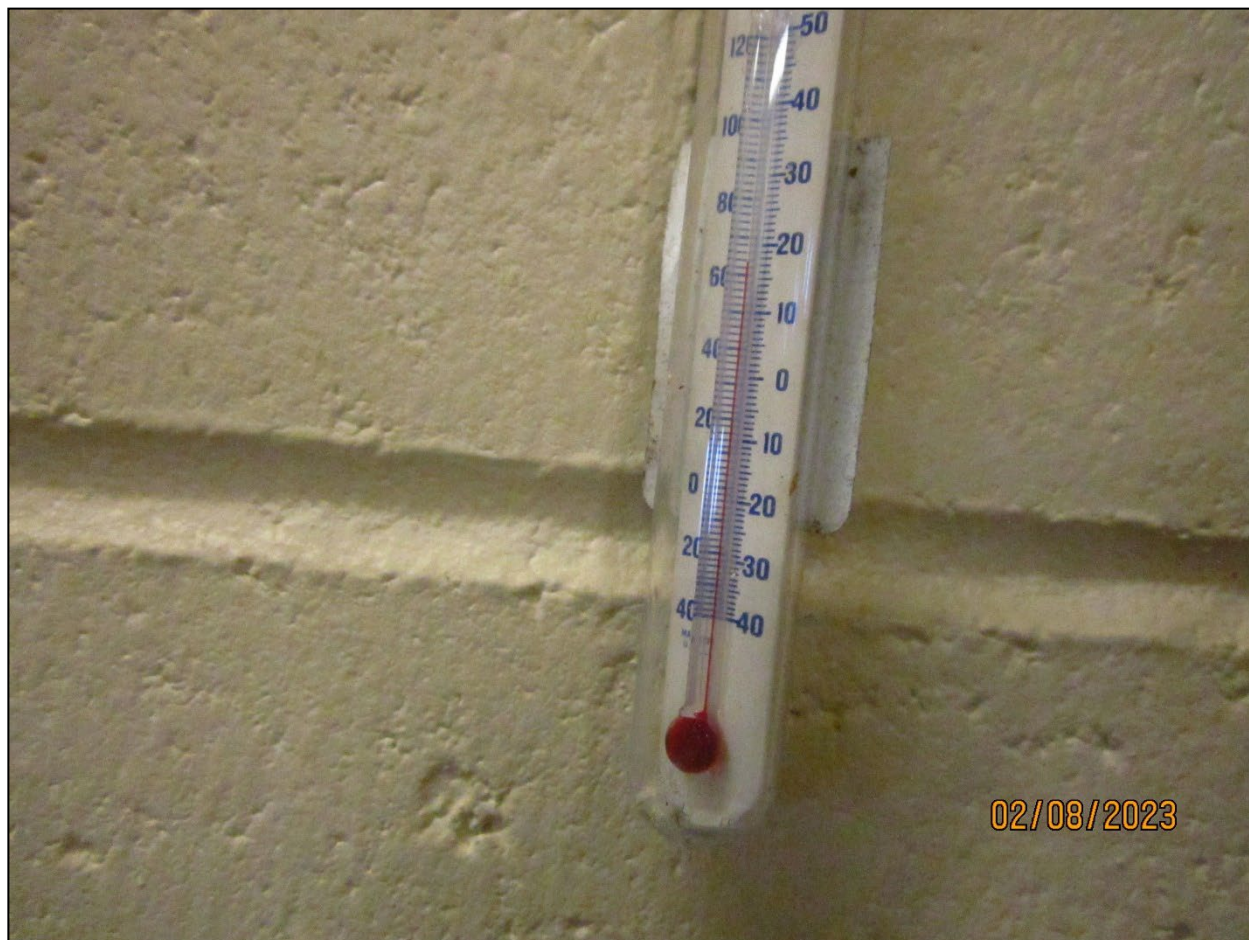
Photograph 33. Thermometer, Sodium Hydroxide Storage/Pump Room View of a thermometer on the wall of the sodium hydroxide room. The thermometer read 64° F.
