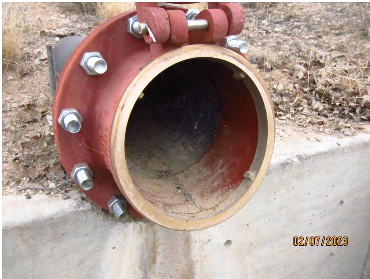
Photograph 19. W0002 Pump-to-Waste Discharge Pipe Opening View of the open W0002 pump-to-waste discharge pipe. The pipe did not contain water, moisture, or debris in the invert.
