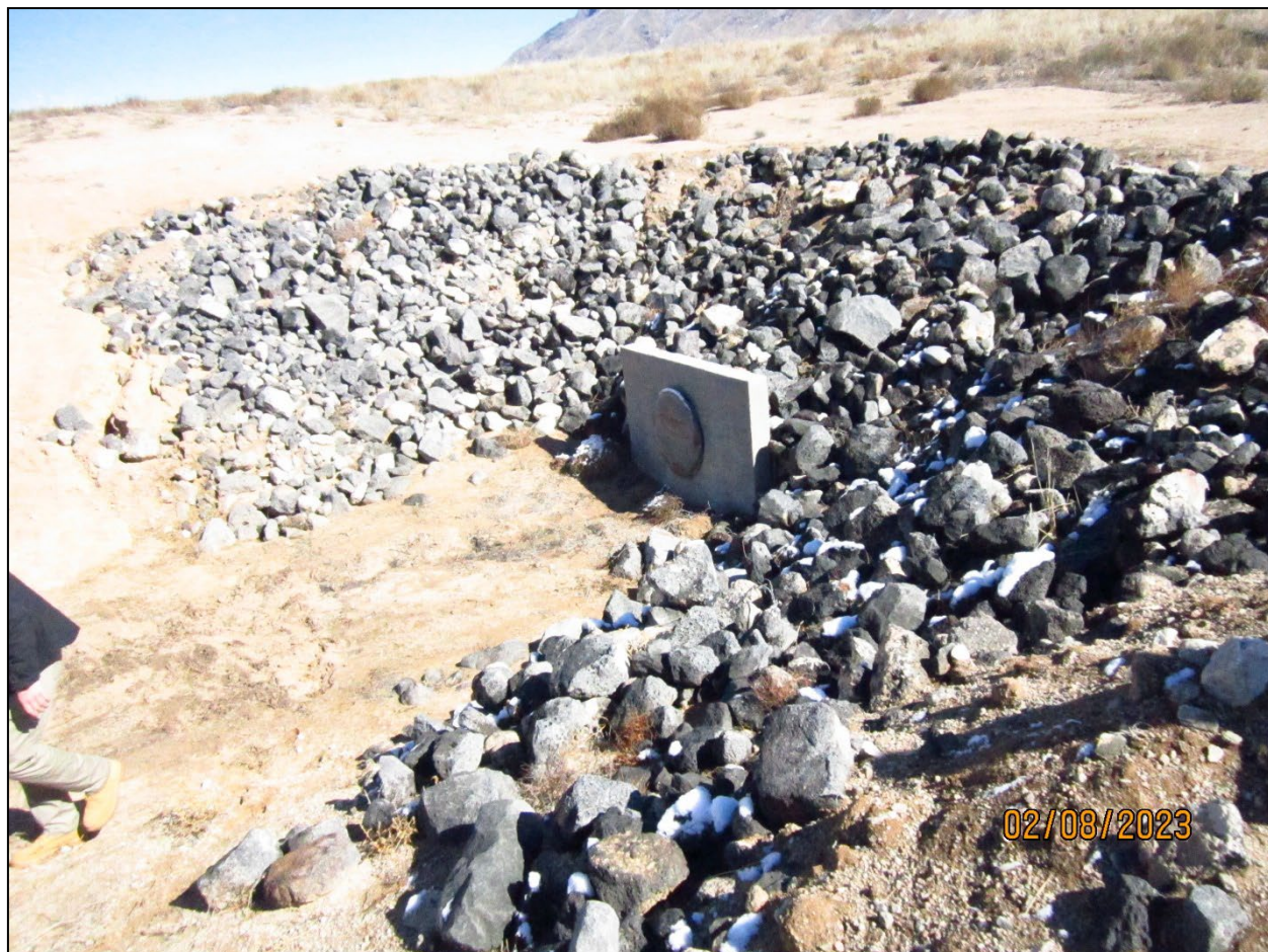
Photograph 60. ST001 Tank Overflow Outfall View of the overflow outfall for the ST001 tank, located approximately 500 feet west of the tank. The opening to the outfall pipe was screened.
