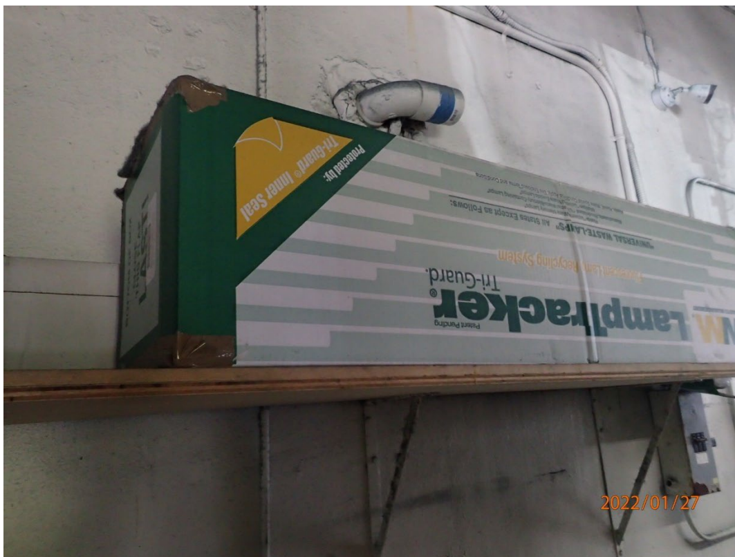
Photo 10: Two cardboard boxes of spent mercury lamps labeled “Universal Waste”, closed, and dated 11/01/2021. CAA1.
