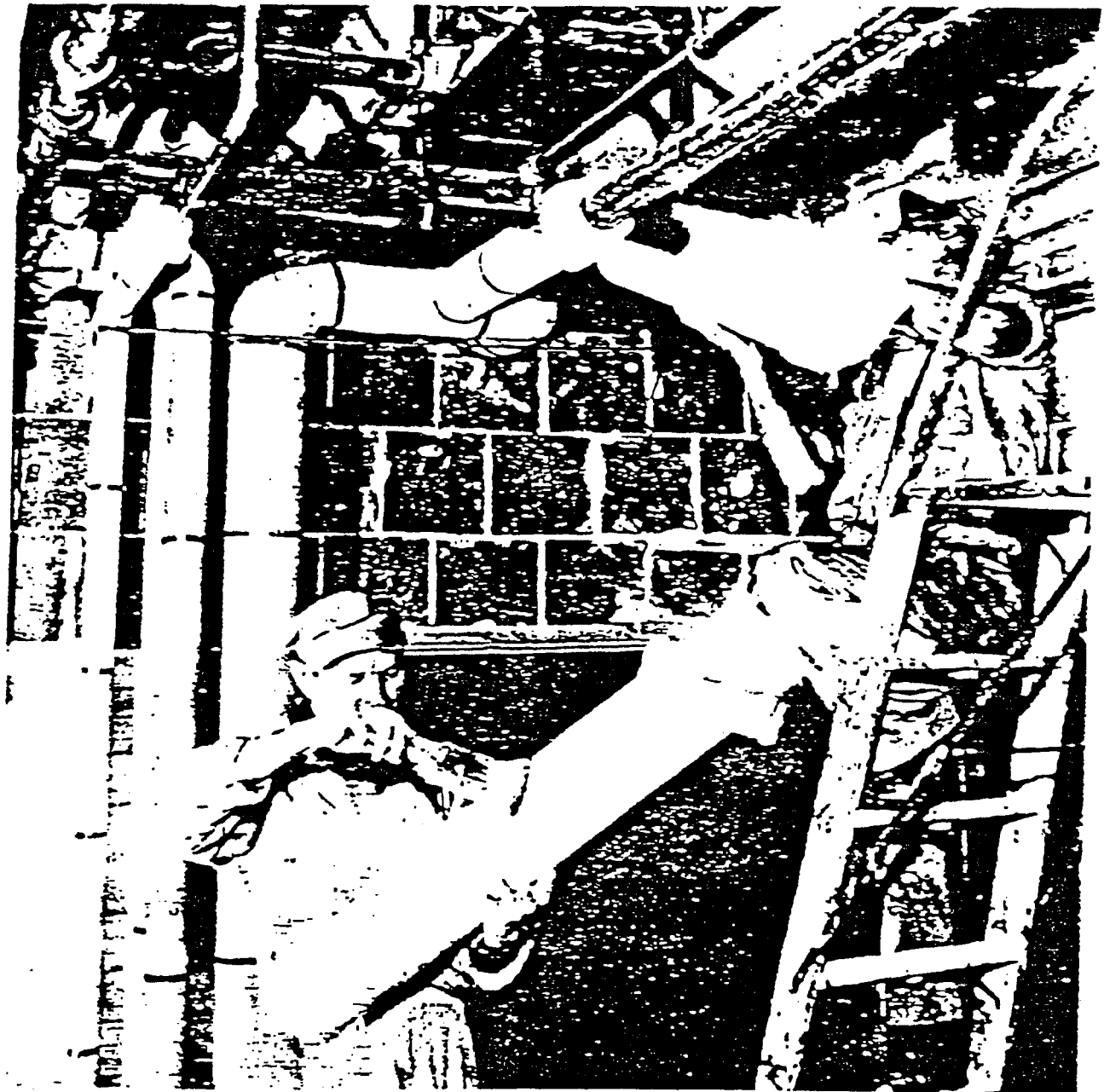
20. Applications of 85% Magnesia pipe insulation are made easily, look neat and clean, last as long as the piping itself.
