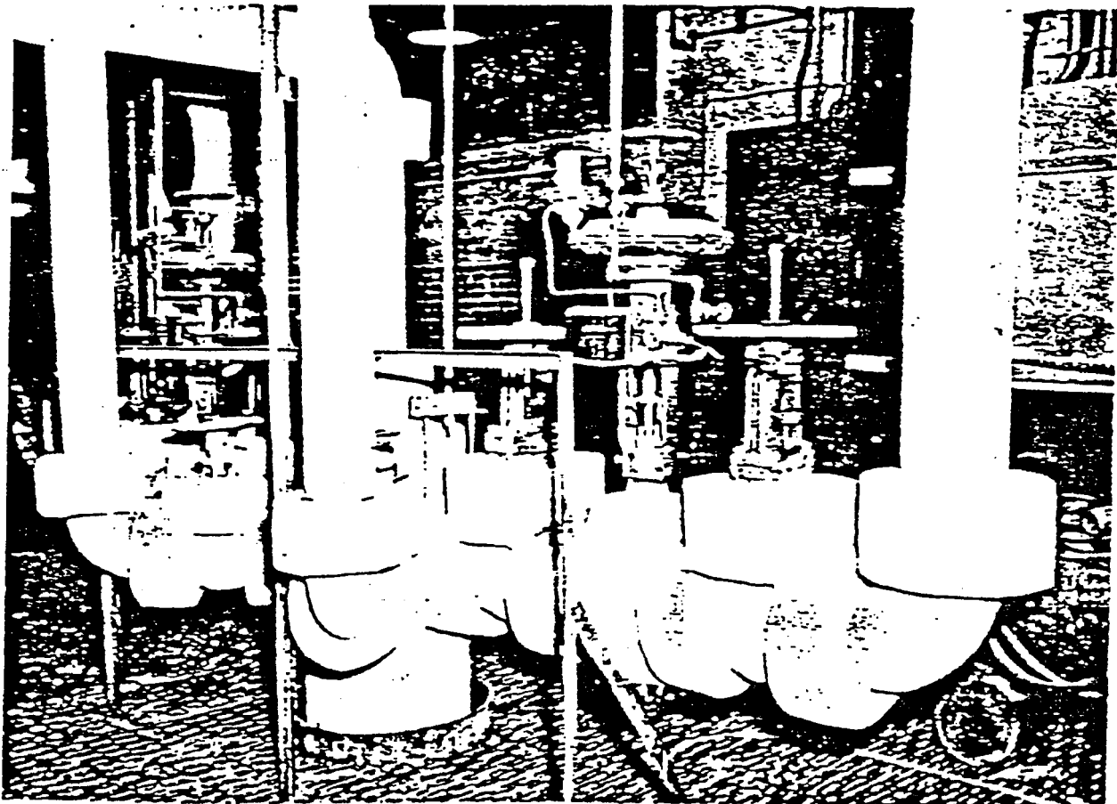
30. Flanges and valves in condensate return piping insulated with 85% Magnesia.
