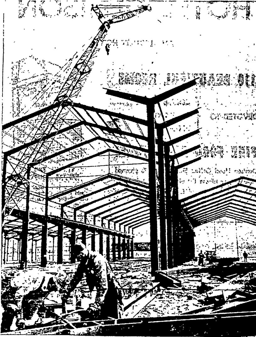
WORKMEN ASSEMBLE a structural steel member that soon will be riveted into the skeleton for one of the seven buildings that will form the backbone of the Johns-Manville Transite pipe plant here.
