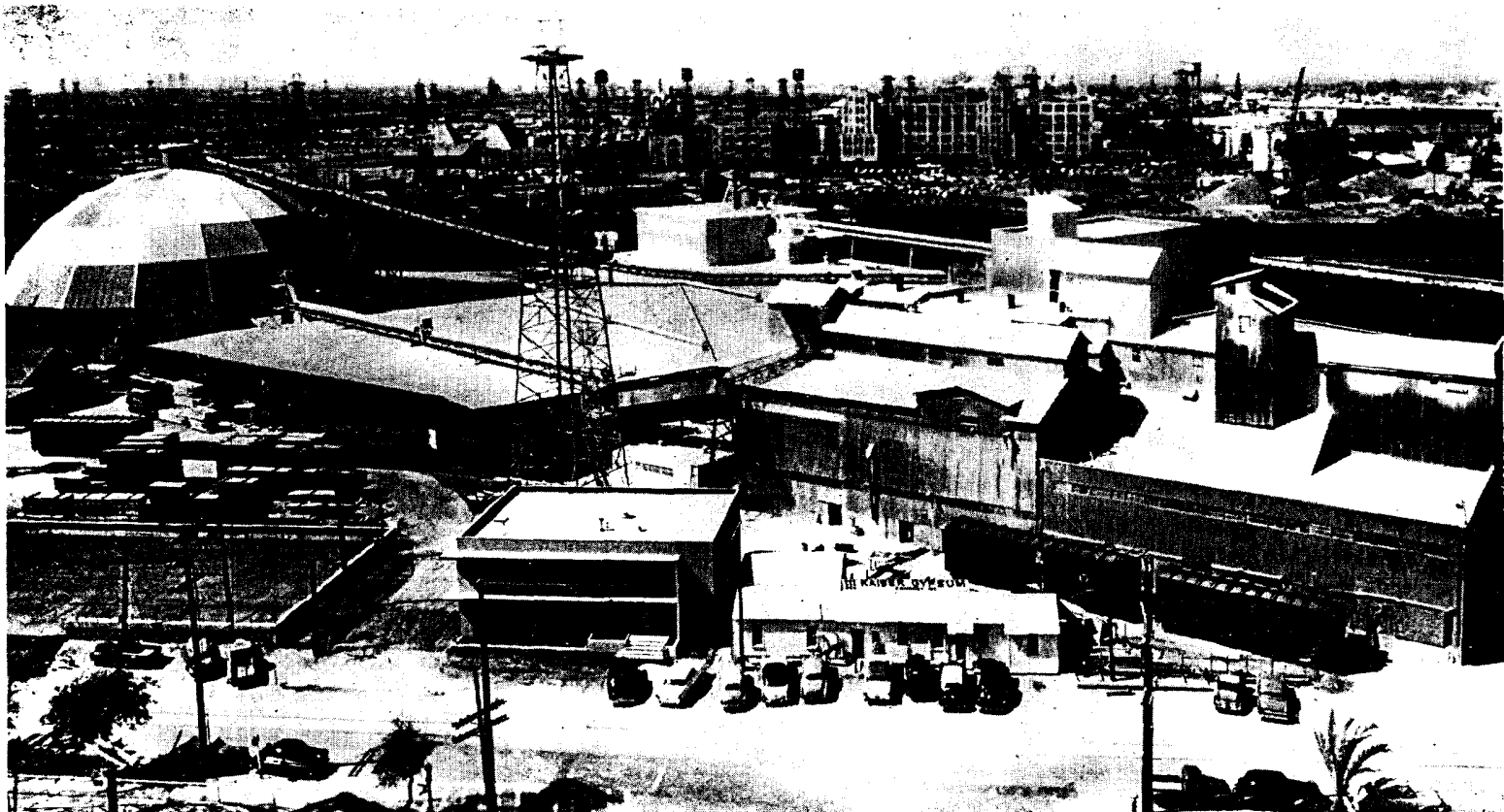
Kaiser Gypsum Company's enlarged Long Beach plant. A 60 per cent expansion just completed increases the facilities annual capacity to 50,000 tons of hardwall and special type plasters and 210,000,000 square feet of gypsum board products.
