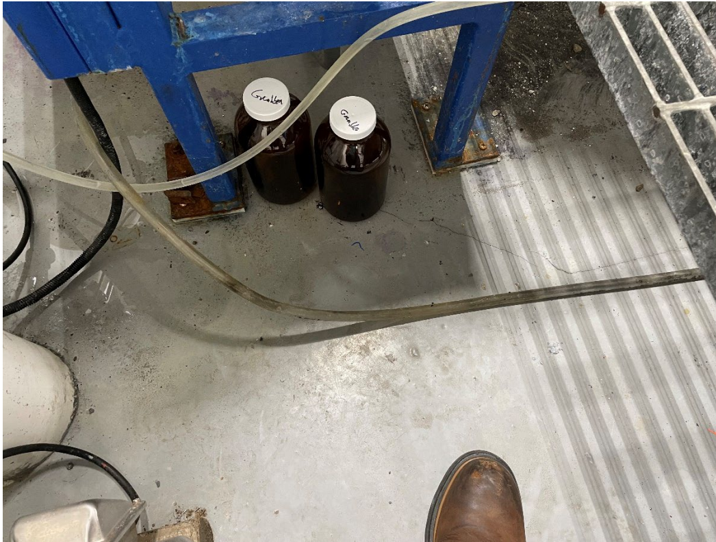
Photo #3. The facility's sample tubing was dirty and/or contain algal growth.
